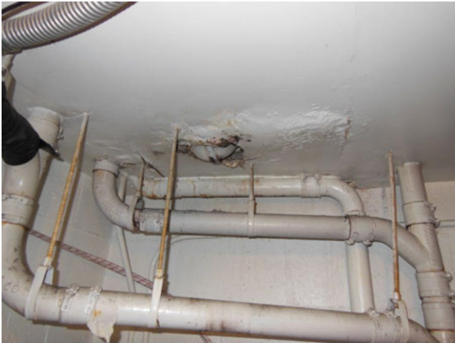
8. Water damaged ceiling in 1<sup>st</sup> floor.
