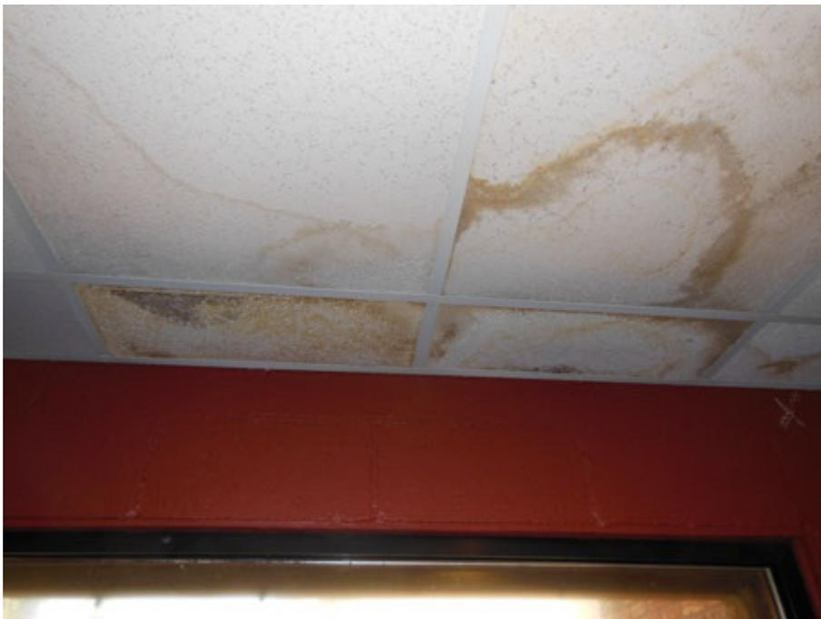
14. Water-stained ceiling panels with mold growth on the 3<sup>rd</sup> floor.
