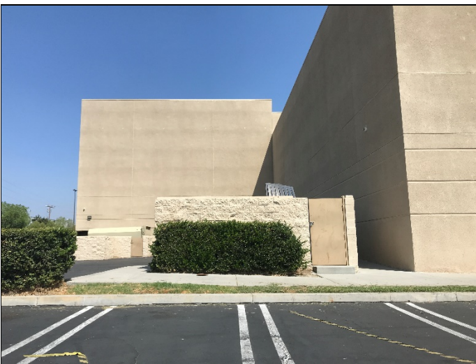
11. Trash Enclosure on the Western Side of the Structure
