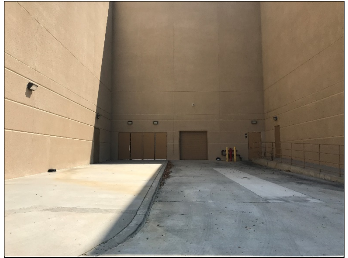
14. Loading Dock on the Western Side of the Structure
