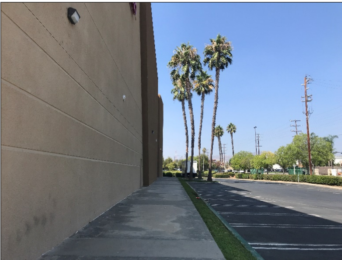
15. The Southern Wall of the Subject Property
