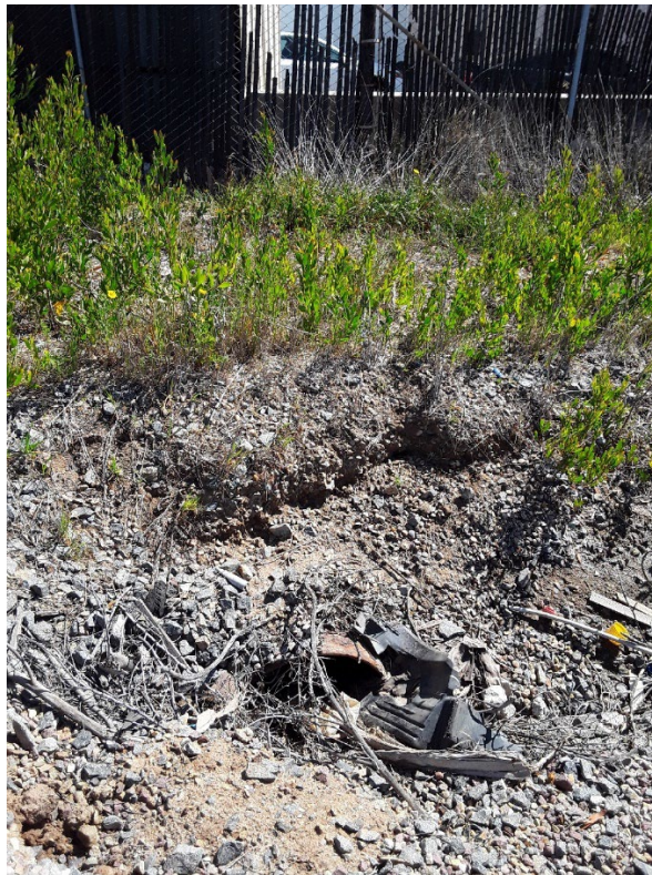
Photo 6. Feature 2 – Culvert adjacent to railroad tracks. March 17, 2022.
