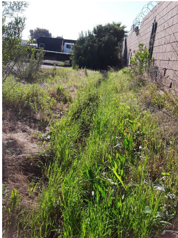
Photo 4. Feature 1 - Manmade brow-ditch, facing south. March 17, 2022.
