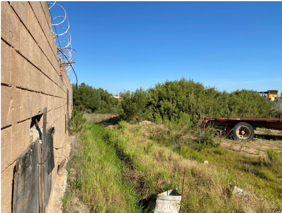
Photo 2. Feature 1 - Manmade brow-ditch, facing north. March 17, 2022.
