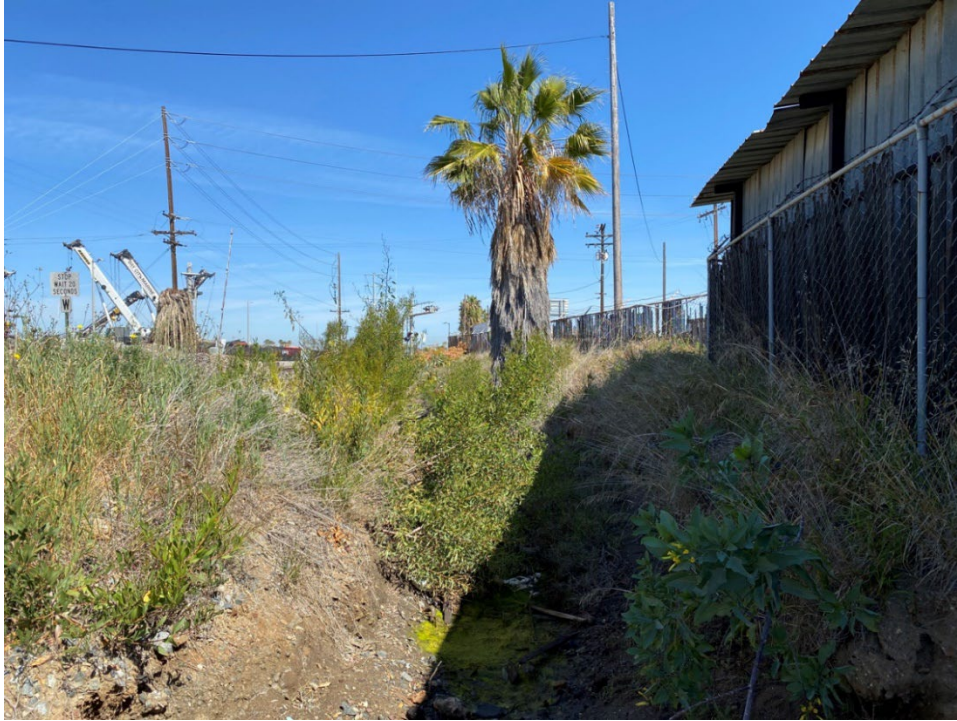
Photo 7. Feature 2 – Manmade brow-ditch upstream of underground crossing, south of Civic Center Dr. and Tidelands Ave. March 17, 2022.
