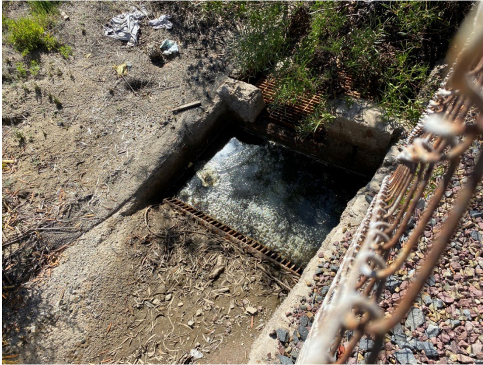
Photo 5. Feature 1 culvert within Remediation Area. March 17, 2022.
