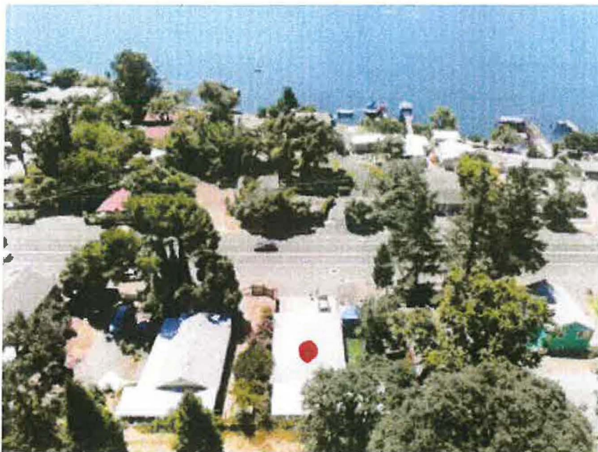
SUBJECT LOOKING SOUTH
