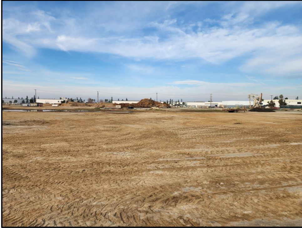
Plate 1: Overview of the subject property, facing south.
