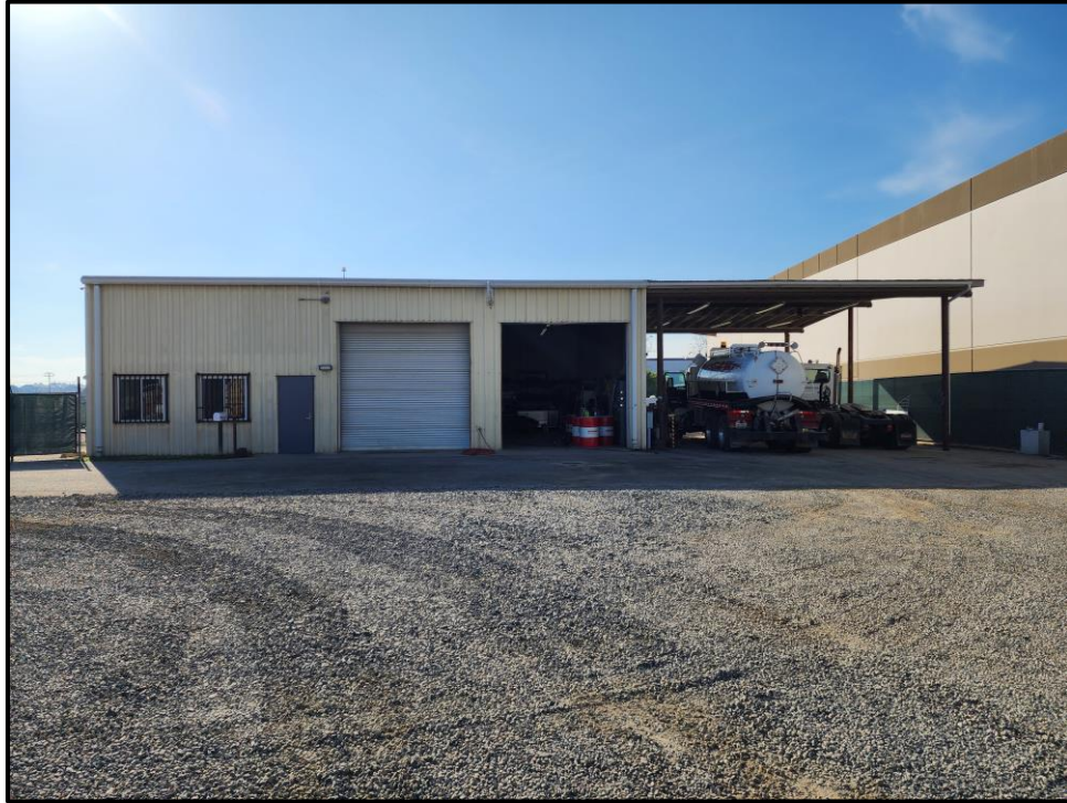
Plate 5: West façade of the main steel building on the property, facing east.
