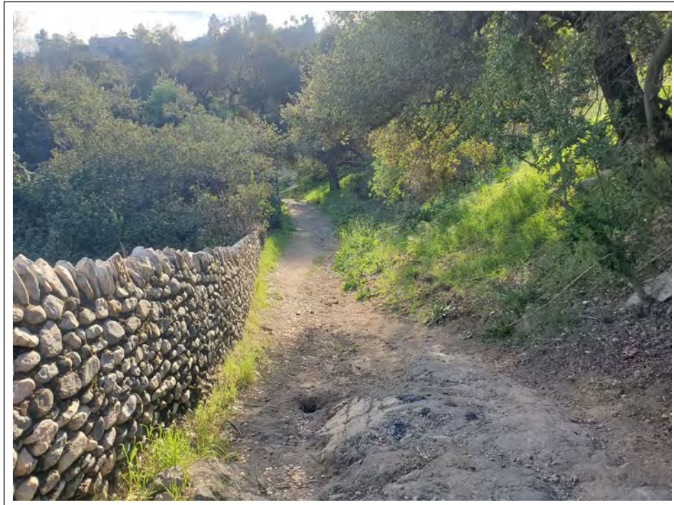
View of the Lower Loop Trail just south of the pedestrian bridge; showing historical boulder retaining wall.
