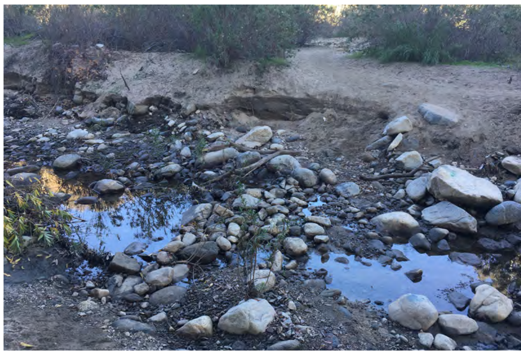
Photo Location 11. January 21, 2022. View of Arroyo Seco in uppermost portion of northern survey area where pedestrians cross the stream.
