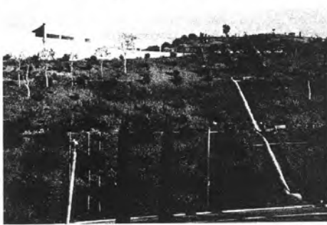
FIG. 2. Conventionally Graded Hill Slope with Planar Face, Rectilinear Drainage Ditch, and uniformly Spaced Plantings
