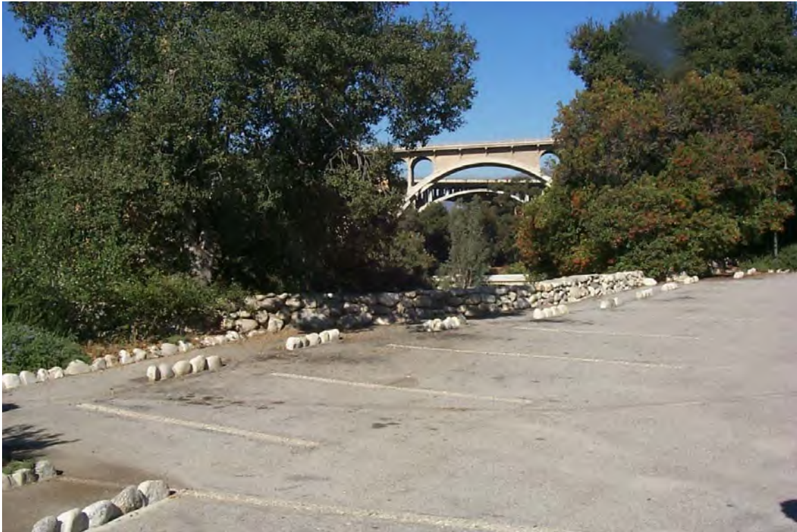
Figure 9-3 Smaller parking areas such as the one above at La Casita are to be encouraged.
