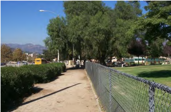
Figure 7-5 While functional, chain link fencing should eventually be removed and replaced by wrought iron or substituted with an arroyo stone wall design solution.
