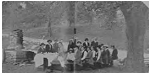
Figure 4-3 A turn of the century “Brookside Breakfast” photo documents traditional recreational use of the Arroyo Seco.
