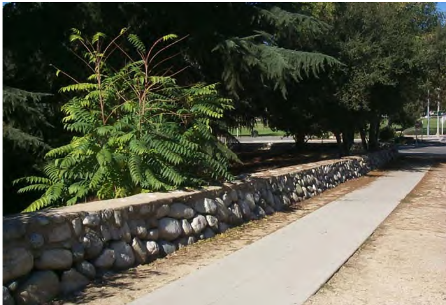
Figure 7-3 This low, well maintained perimeter wall is multifunctional, setting an open, friendly border to the park and offering a sitting space for the park user.
