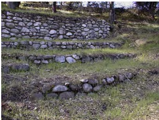
Figure 11-7 Amphitheatre seating is in need of repair.
