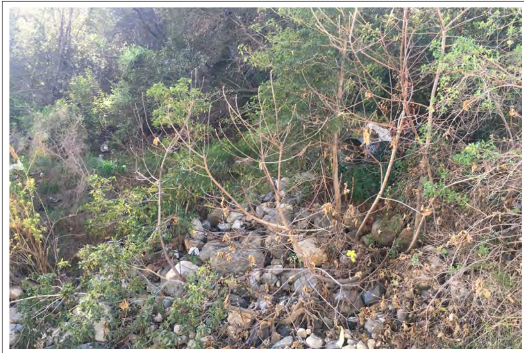
Photo Location 9. January 21, 2022. View of Feature D. A metal pipe that likely drains nearby roads can be seen among vegetation in background.
