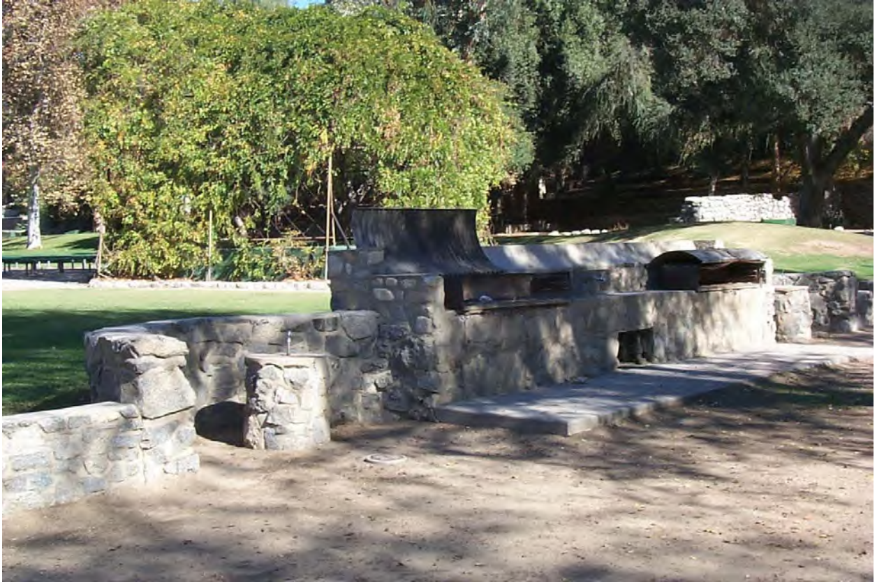
Figure 11-10 Existing arroyo stone grill areas can be custom converted into improved facilities by replacing grill surfaces with a comparable standard model insert.
