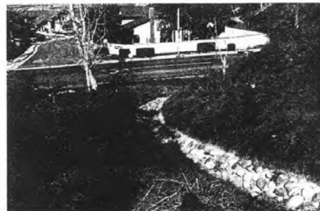
FIG. 5. Example of Landform Grading with Drainageway that is Placed in Special Swale-and-Berm Combination to Conceal it from View
