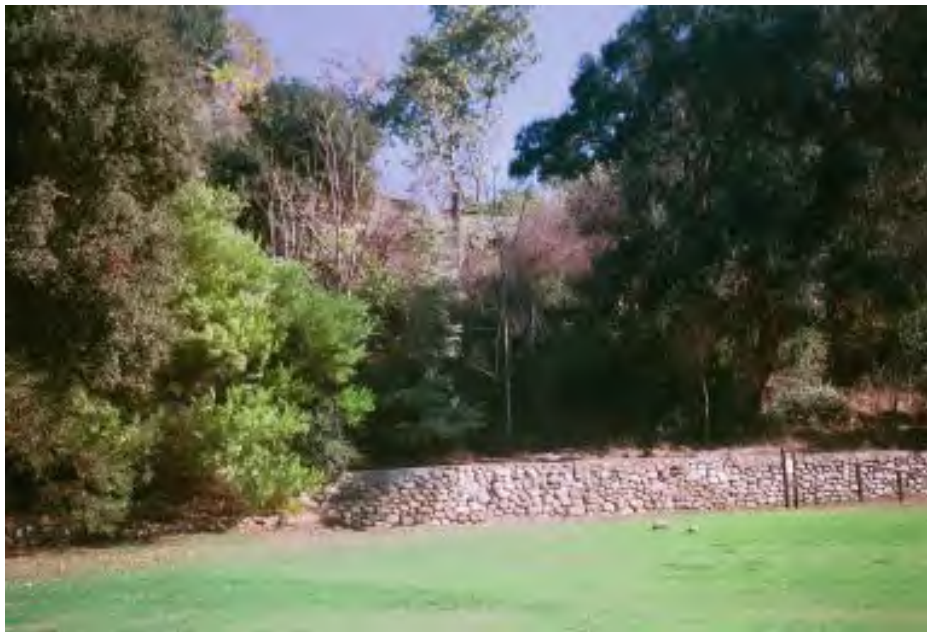
Figure 7-4 The natural materials of the perimeter walls blend well with open space areas of the park.
