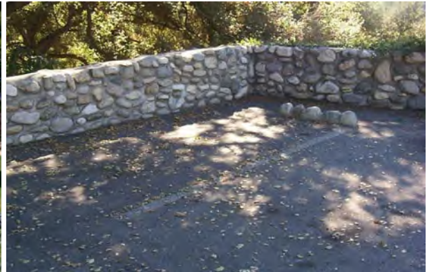
Figure 7-6 This type of low, arroyo stone interior wall is to be emulated in future park improvements.
