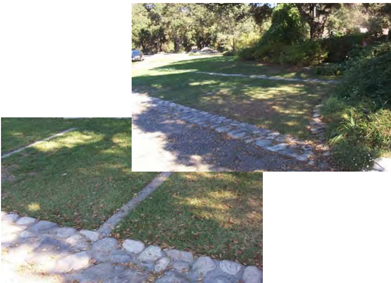
Figure 9-8 Specialized parking stalls here are a good example of balancing parking needs with the natural environment.
