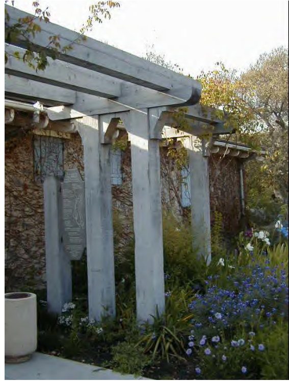
Figure 3-5 The trellis structure at La Casita in Lower Arroyo is a good example of heavy timber construction.
