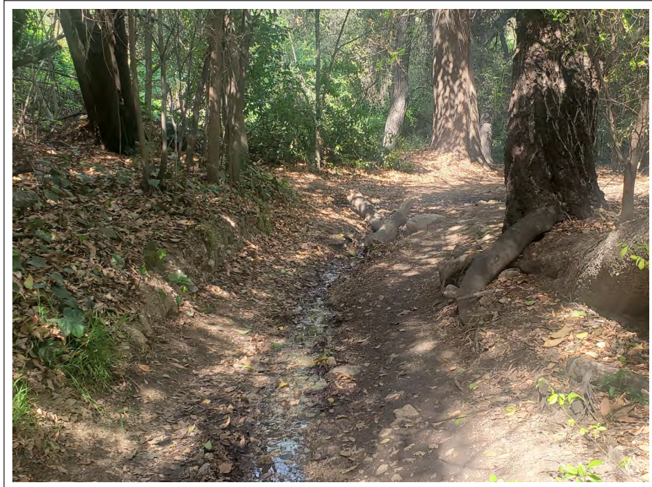
View of a drainage area along the Upper Loop Trail.
