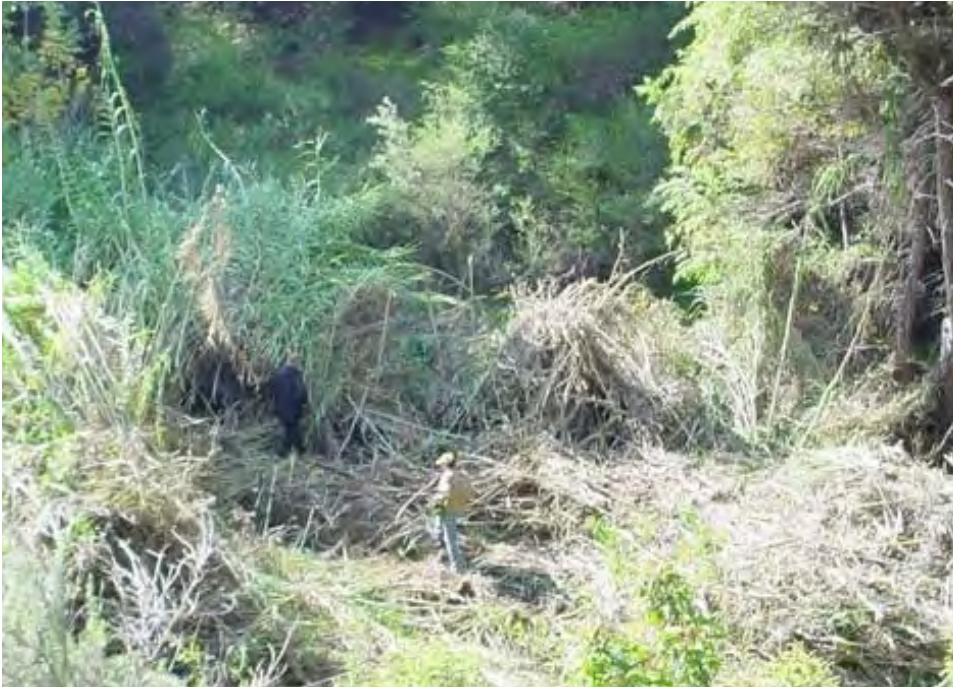
Figure 2-10 Brush clearing shall be balanced with habitat conservation and slope protection.
