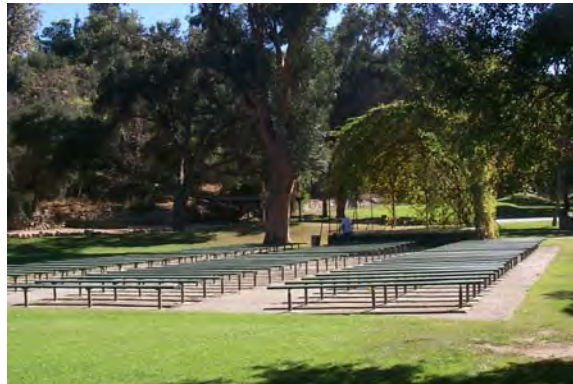
Figure 11-8 Seats and stage structure are in need of repair at the stage area in Brookside Park.
