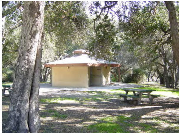
Figure 3-4 Existing Restroom in the Oak Grove upper Arroyo Seco
