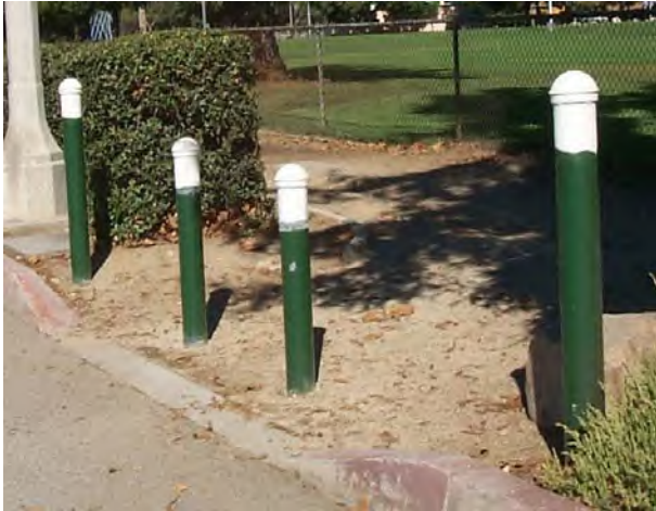
Figure 9-4 White capped bollards help to control regular vehicular access while still allowing passage by pedestrians.
