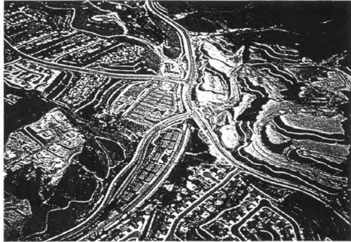
AERIAL PHOTO of landform-graded region in Anaheim Hills. Note irregular patterns formed by landform-graded slopes along perimeter of lot pads.
