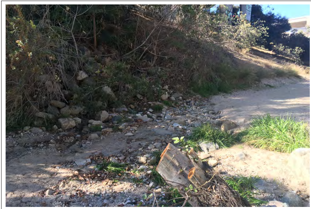
Photo Location 9. January 21, 2022. View of area where water that comes out of Feature D pipe crosses the trail and causes minor erosion.
