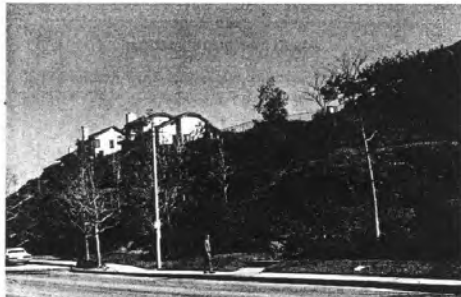
FIG. 6. Example of Landform Grading and Revegetation with Concave and Convex Slope Forms and Nonlinear, Varying Slope Gradients
