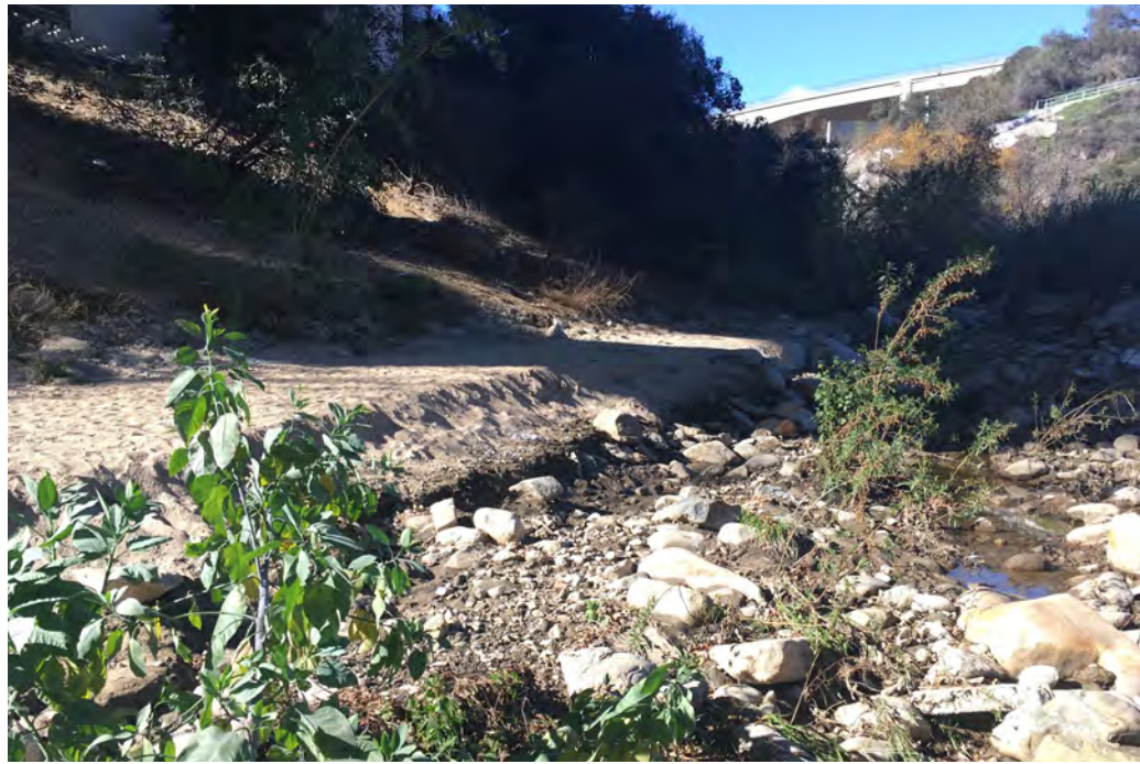
Photo Location 10. January 21, 2022. View of the relation between the trail under the freeway bridge and the adjacent Arroyo Seco. Shelving along bank can be seen that indicates the level of the Ordinary High Water Mark.
