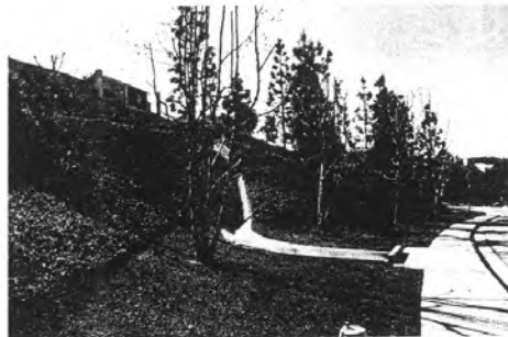
FIG. 16. Landform-Graded Slope with Convex and Concave Slope Shapes, Varying Gradient, Curvilinear Drainage Ditch Concealed in Berm and Swale Configuration, and Clustered Plantings
