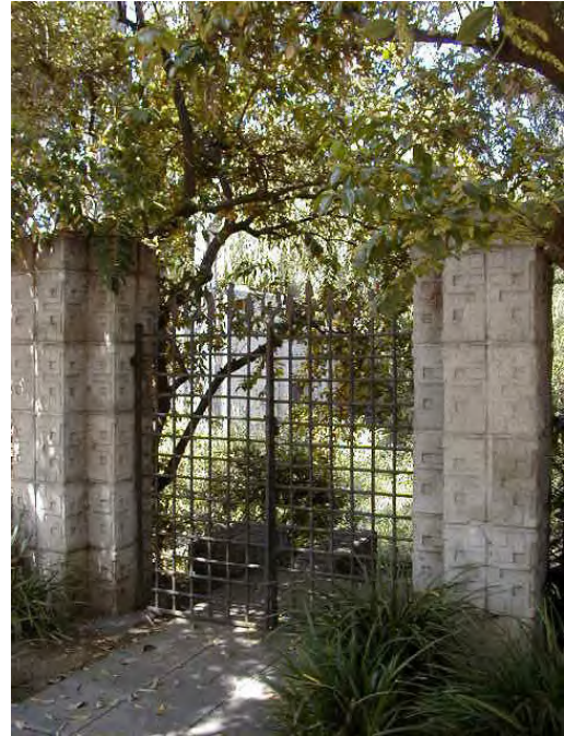
Figure 7-1 The neighboring residential gates along the Arroyo Seco offer excellent examples of appropriate design.
