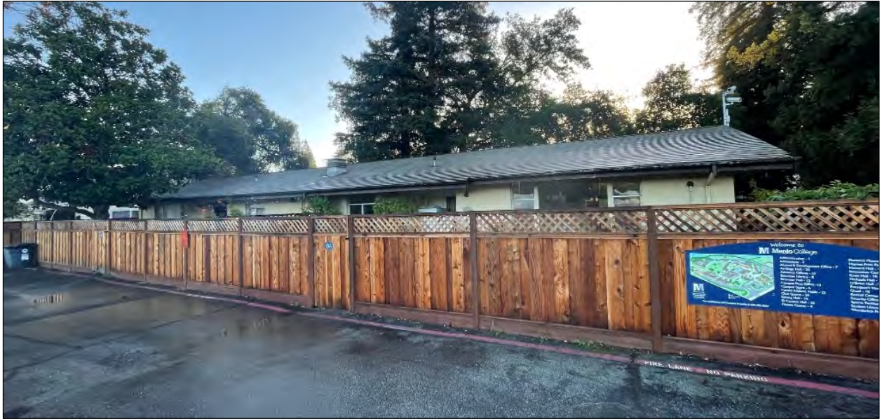
Front Entrance - View facing East
