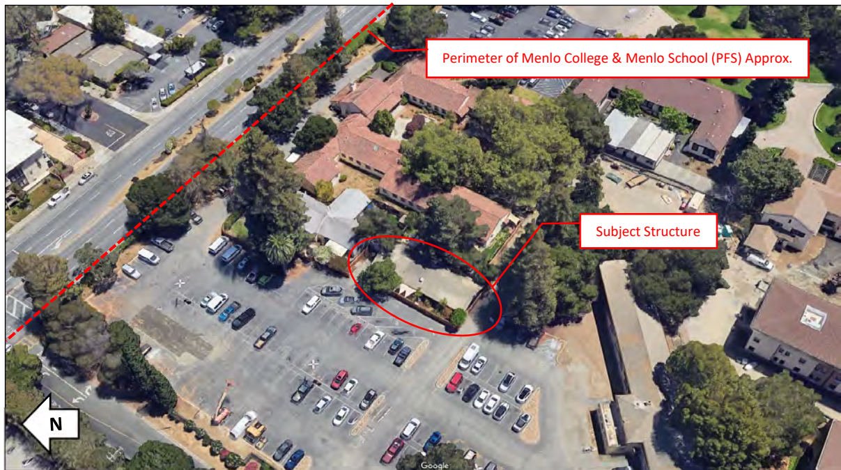
Figure 2: Subject Structure Aerial View. Source: Google Maps, 2024.
