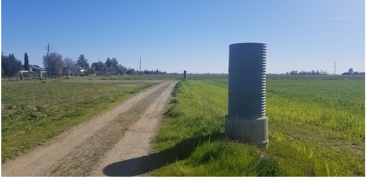
Overview of Project area from second riser along access road, facing east. Project cell tower pad will be adjacent to riser at the end of the access road in the center of the photo. Underground utility easement will extend from tower location northeast to the power pole with transformer at right in the photo.
