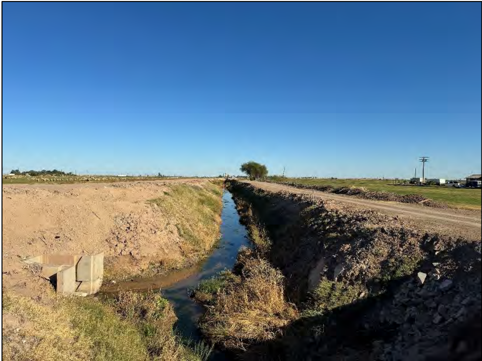
Figure 11. Northern portion of Acacia Five A Drain in Project Area, facing south
