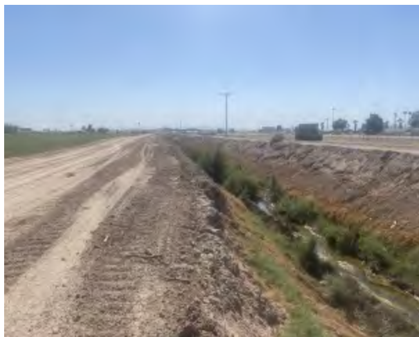
Photo 12 Comments: Another view of the drainage ditch to the w of the Subject Property looking S.
