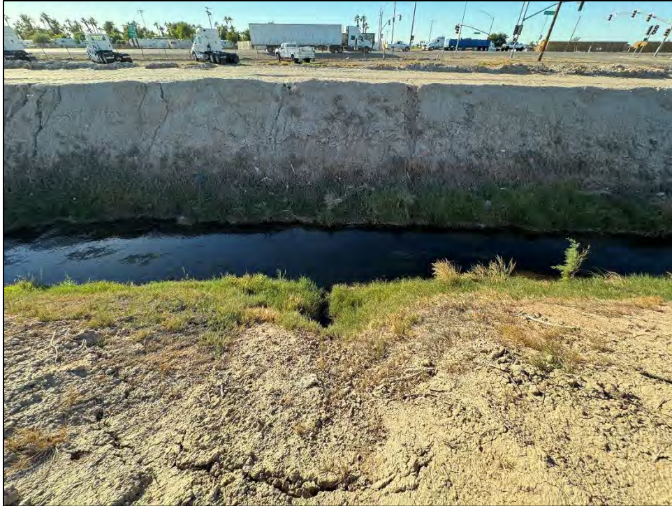
Figure 12. Side wall of Acacia Five A Drain, facing west
