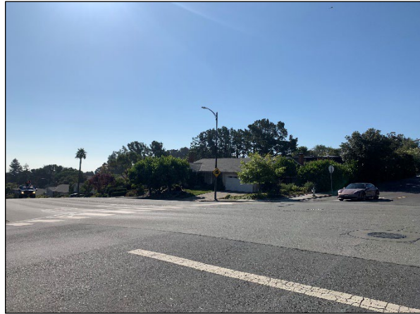
Photo taken proposed pothole location 5, facing southeast.
