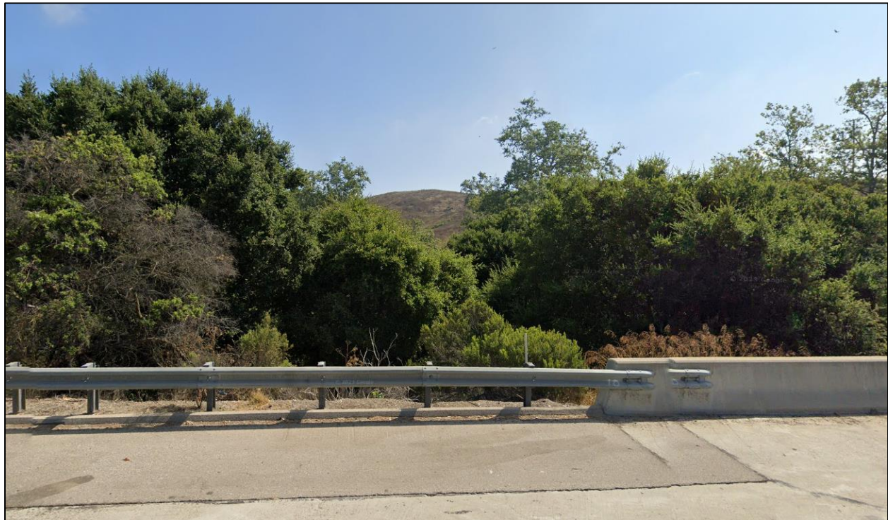
FIGURE 3. VIEW OF PROJECT SITE TRAVELING NORTHBOUND ON HIGHWAY 101. WORK AREA IS AT GROUND LEVEL WHILE THIS SECTION OF THE HIGHWAY IS ELEVATED TO ALLOW DOS PUEBLOS CREEK TO FLOW UNDERNEATH.
