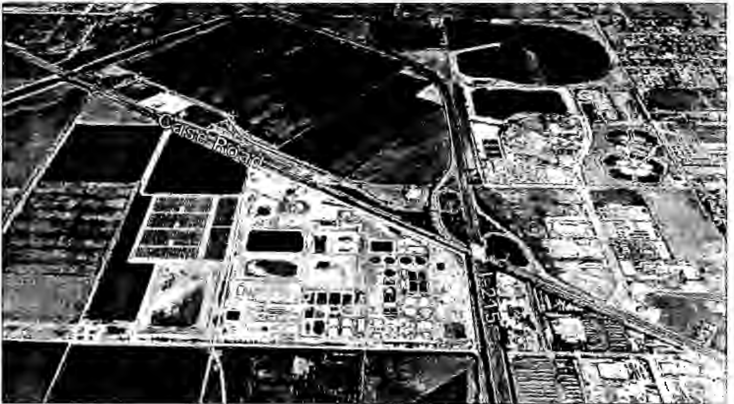
Perris Valley Regional Water Reclamation Facility
