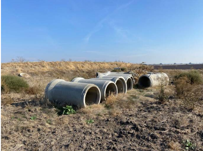
7. Stormwater pipe on south central portion of the Subject Property.
