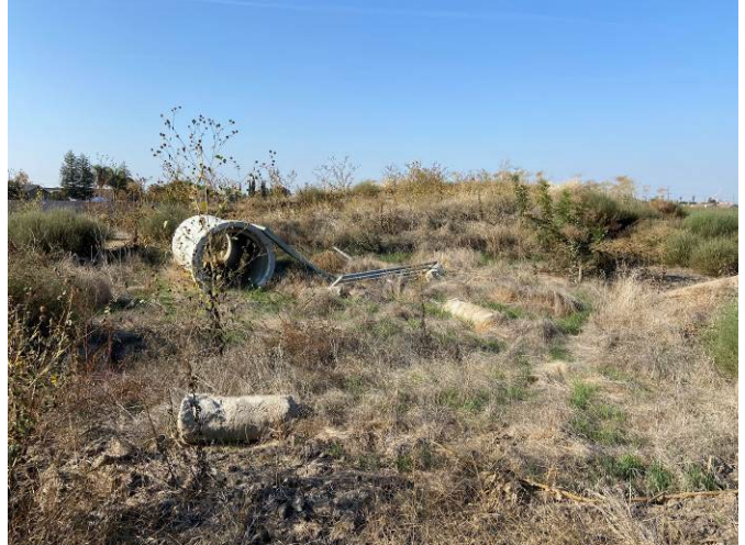
8. Stormwater pipe at east side of the mounded soil of Photograph 6.
