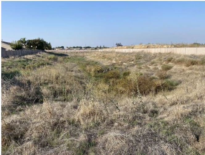
5. Stormwater basin on southeast portion of the Subject Property.
