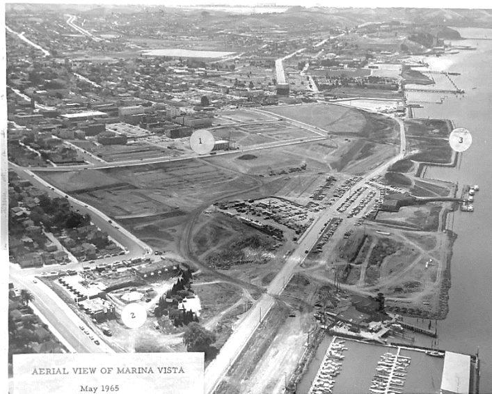
Aerial View of the Marina Vista Redevelopment Project Under Construction, Facing Southeast, May 1965. The extant ferry basin and the former Mare Island Ferry terminal are visible in the right middle ground (below the circular marker labeled "3"). Source: Vallejo Naval and Historic Museum.
