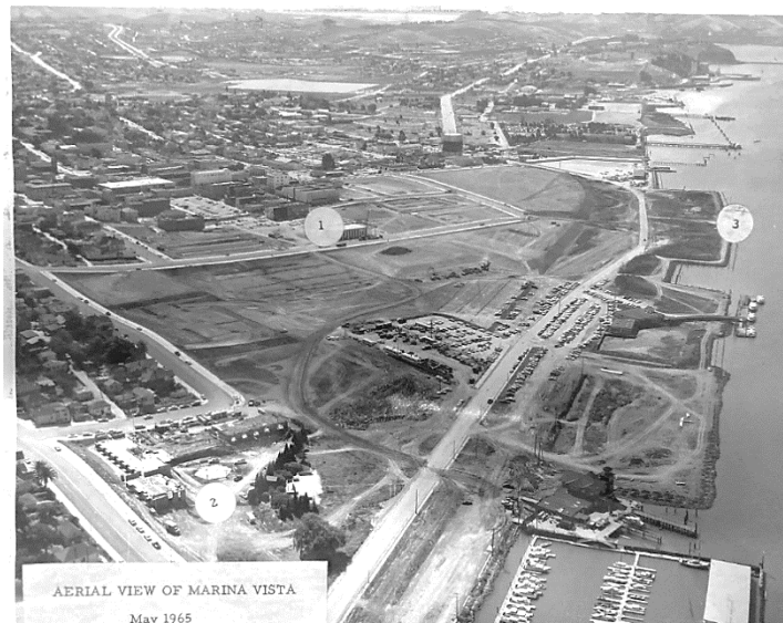
Aerial View of the Marina Vista Redevelopment Project Under Construction, Facing Southeast, May 1965. The extant ferry basin and the former Mare Island Ferry terminal are visible in the right middle ground (below the circular marker labeled "3"). Source: Vallejo Naval and Historic Museum.
