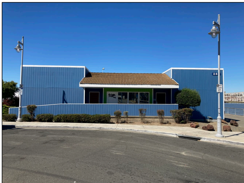
P5b. Description of Photo: View of primary (northeast) façade, facing southwest. ESA, 2023.
