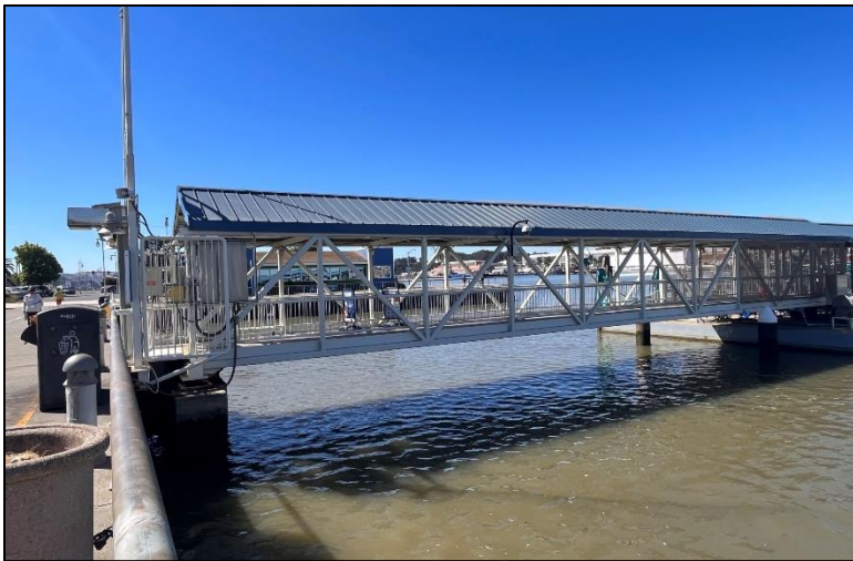
Photo 6: Existing ferry terminal infrastructure. Photo taken on July 25, 2023 facing southeast.
