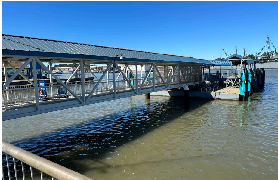
Existing Vallejo Ferry Terminal gangway and float.
