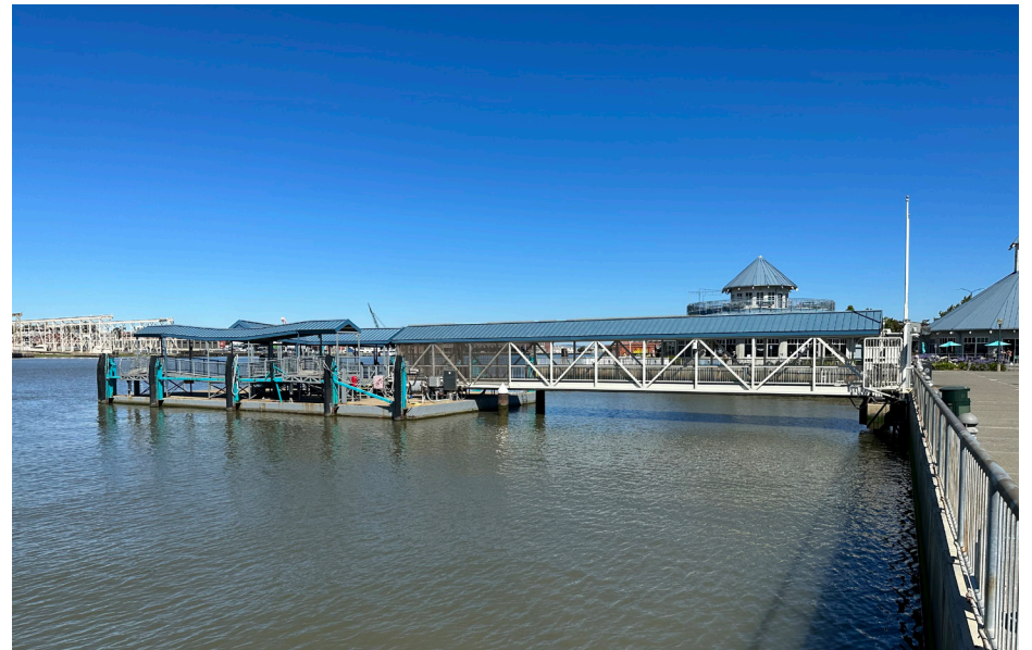
View of existing Vallejo Ferry Terminal facing north.
