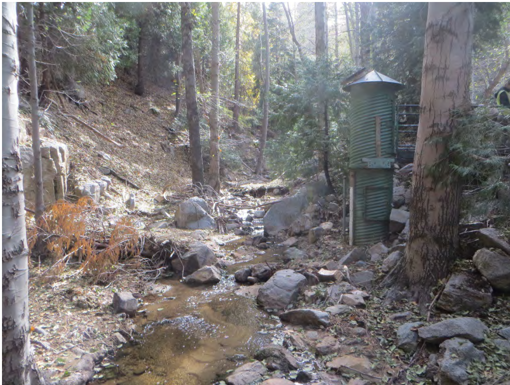
Photograph 10: From an area inside Houston Creek, which runs adjacent to the proposed project site, looking south upstream toward Lake Gregory Dam.
