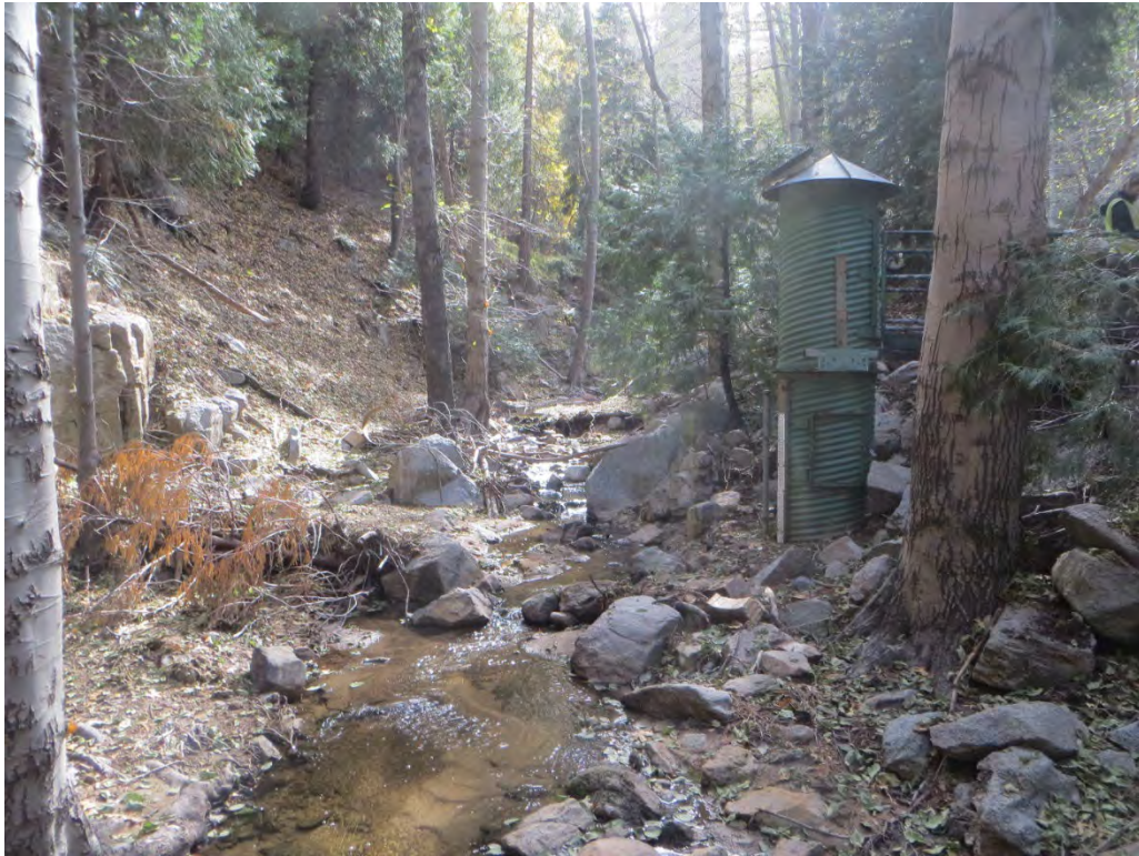
Photograph 5: From the middle of Houston Creek, looking south upstream at the existing riser and footbridge which extends from the eastern boundary of the project site.
