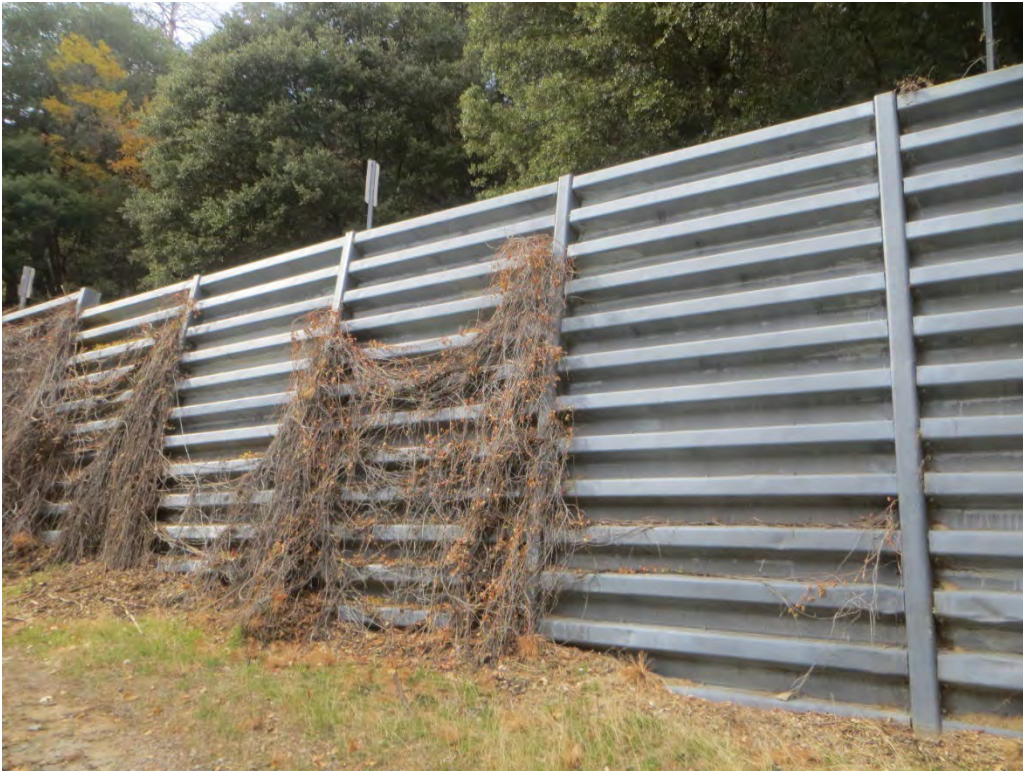
Photograph 1: From the inside the project site, looking west at a guard rail marking the eastern boundary of Houston Drive and the existing sewer main line.
