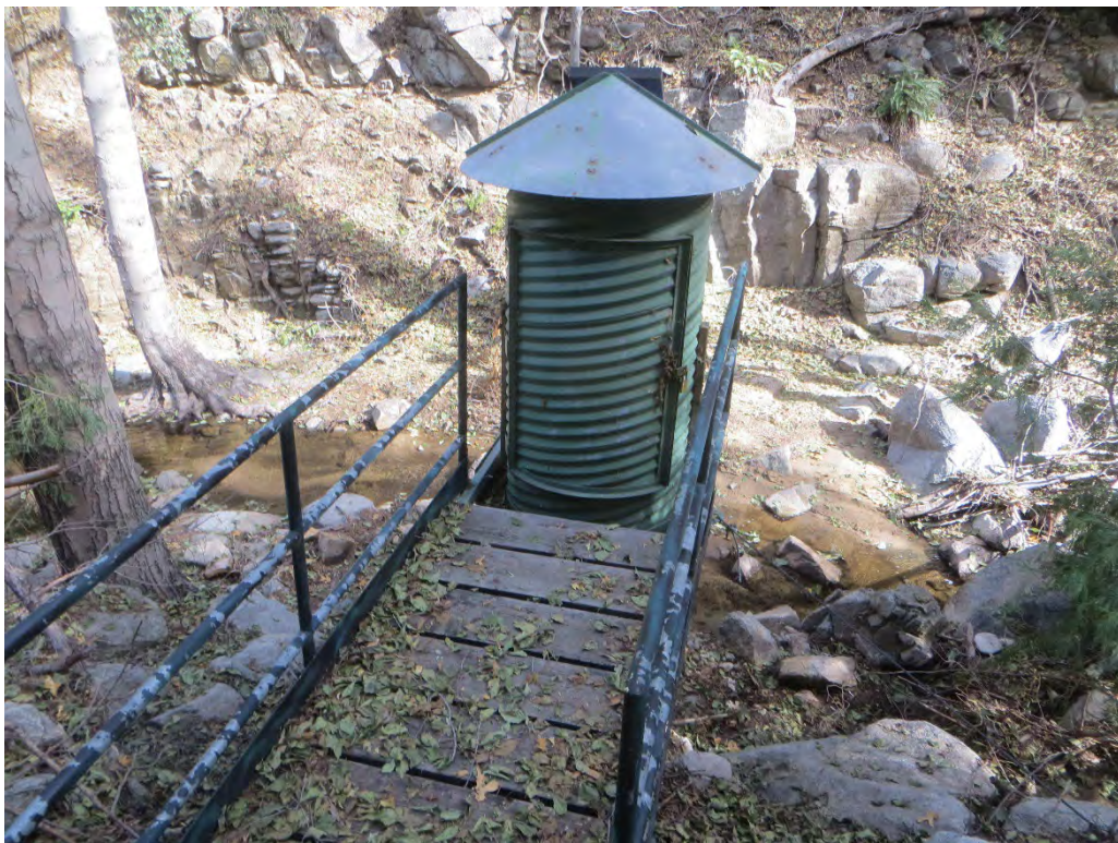
Photograph 4: From the eastern boundary of the project site, looking east at an existing riser and footbridge along the western bank of Houston Creek.
