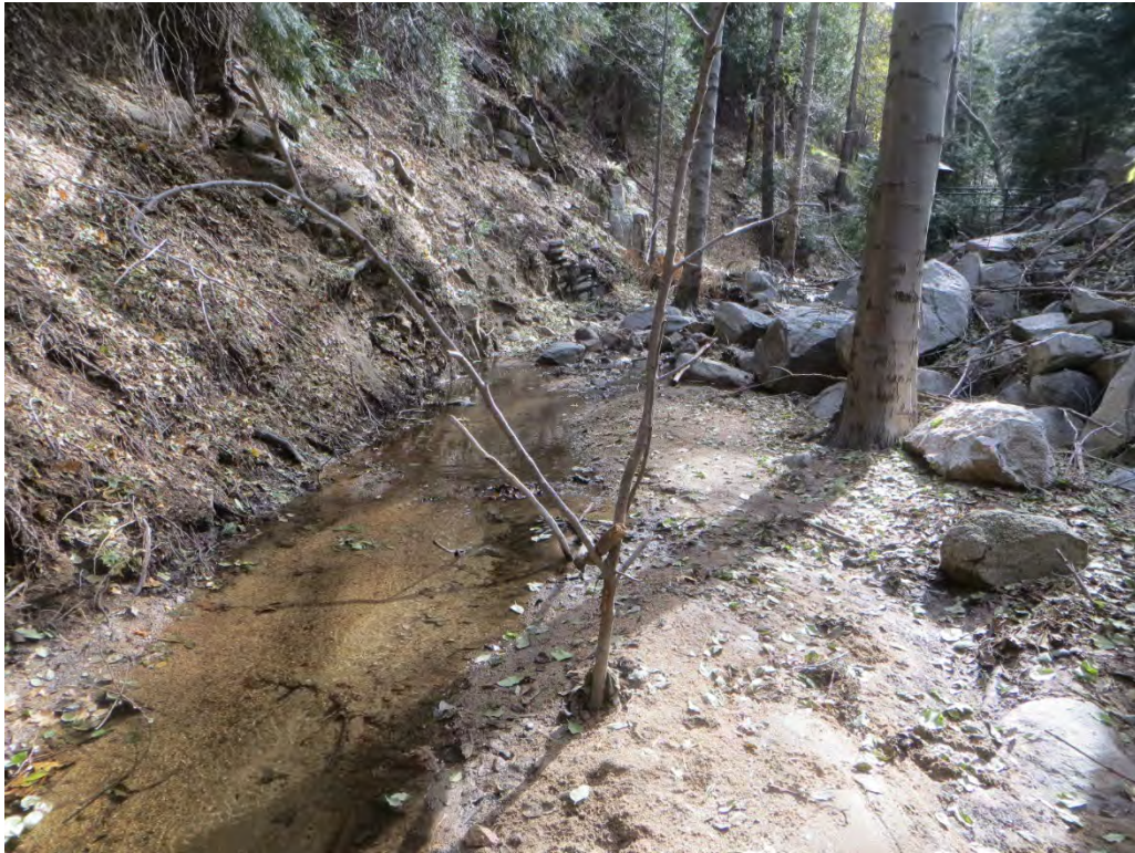
Photograph 7: From the middle of Houston Creek, looking south upstream through supported vegetation.
