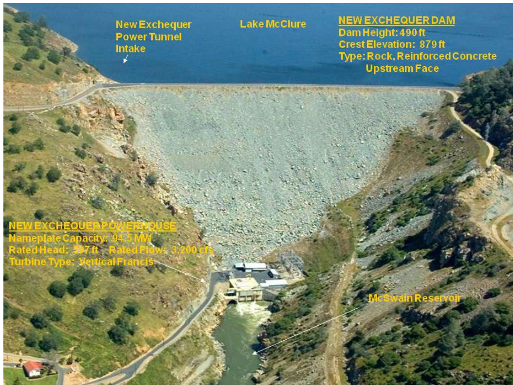
Figure 1-2. New Exchequer Powerhouse
