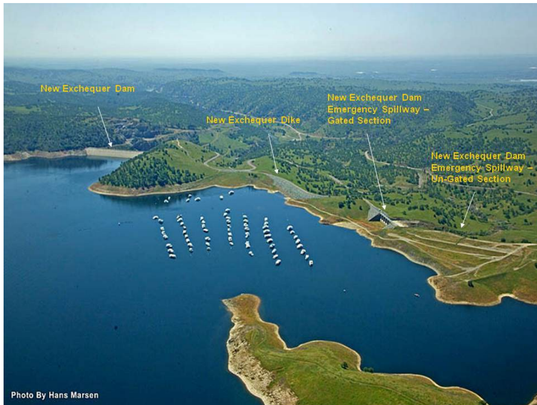
Figure 1-1. New Exchequer Dam and Hydropower Facilities
