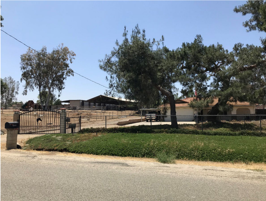
Site 5 – James Amer (Residential Property) (18765 Markham St, Riverside, CA). Photo facing northwest.
