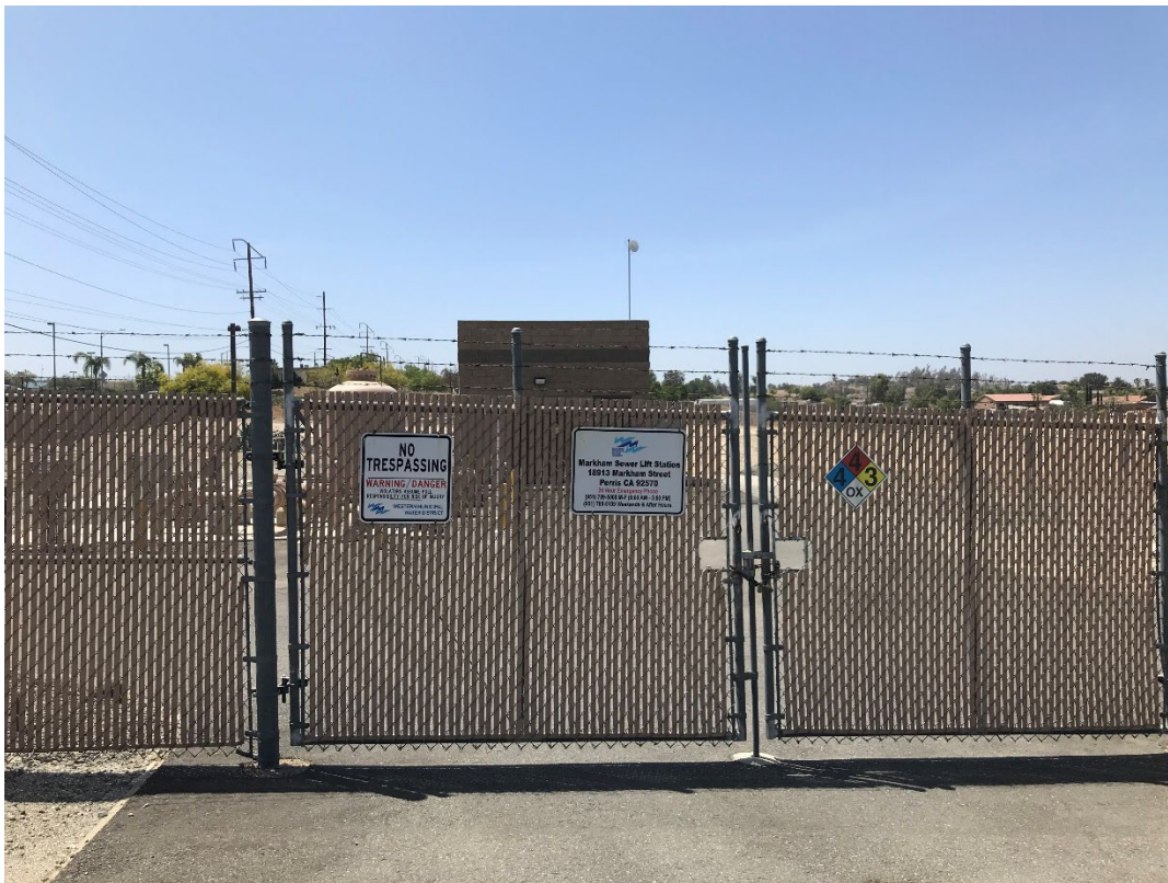
Site 8 – Markham Sewer Lift Station (18913 Markham St, Perris, CA). Photo facing south.
