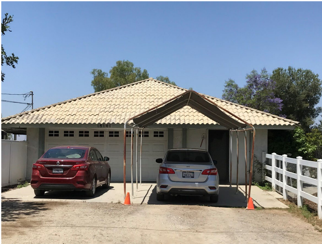
Site 2 – Randy Peek (Residential Property) 18141 Birch Street, Perris, CA). Photo facing west.
