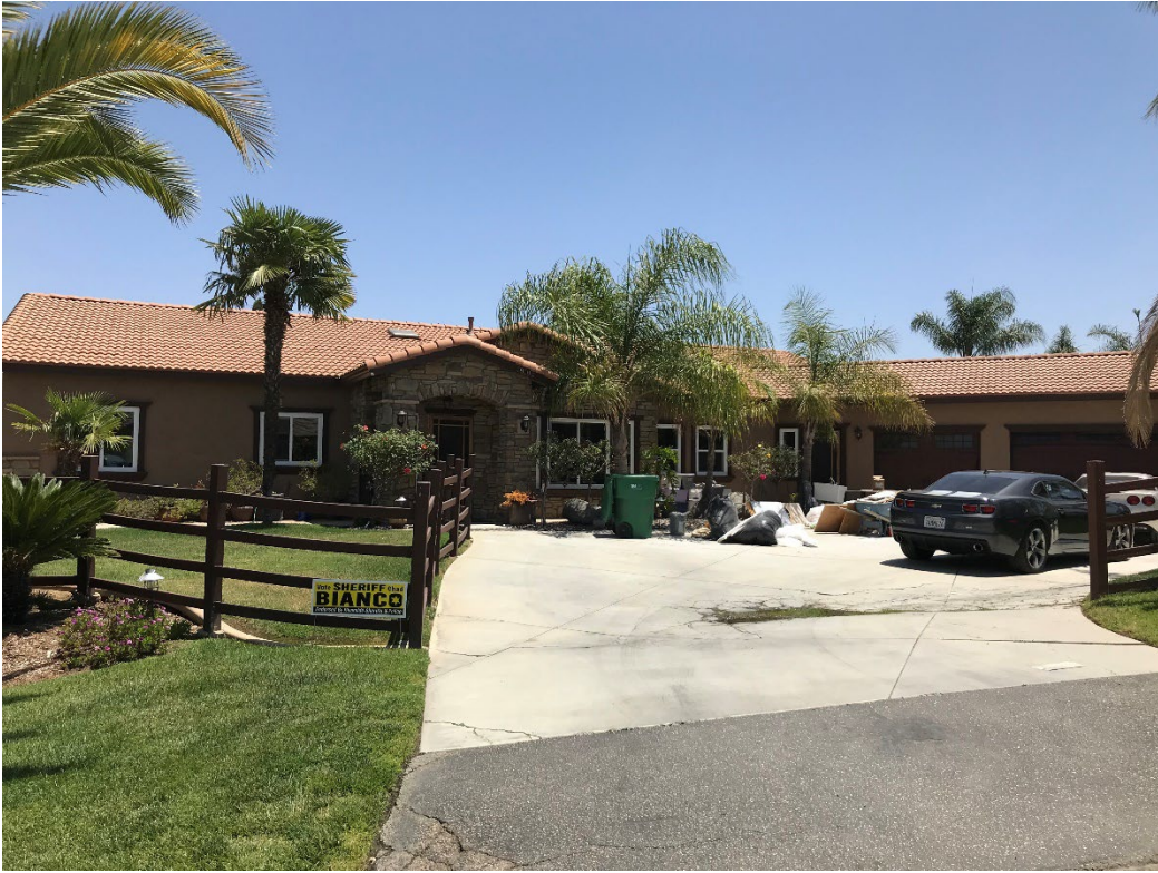
Site 6 – AZ Crane, Inc. / Kelly Zamora (Residential Property) (18194 Andrew Ct, Perris, CA). Photo facing east.
