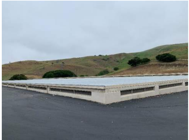
Looking at the reservoir from the southwest corner of the Project site with open space in the background.
