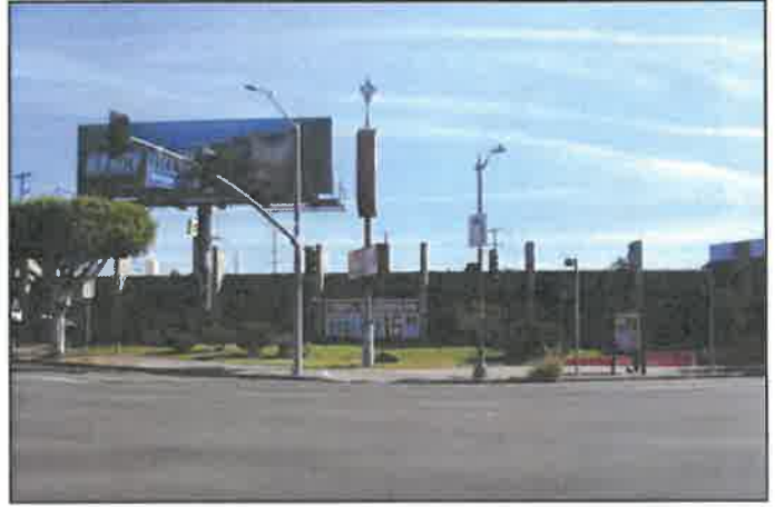
View 2: On the southwest corner of Hollywood Blvd and N. Vermont Ave, looking northeast at the Project Site.
