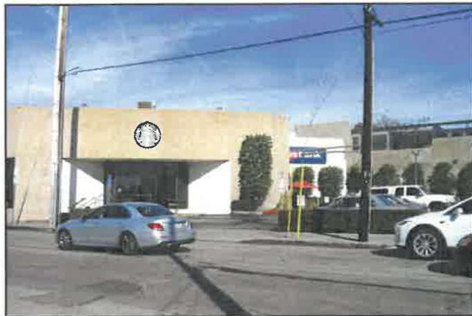
View 11: On the south side of Prospect Ave, adjacent to the alleyway, looking northwest at the commercial properties north of the Project Site.
