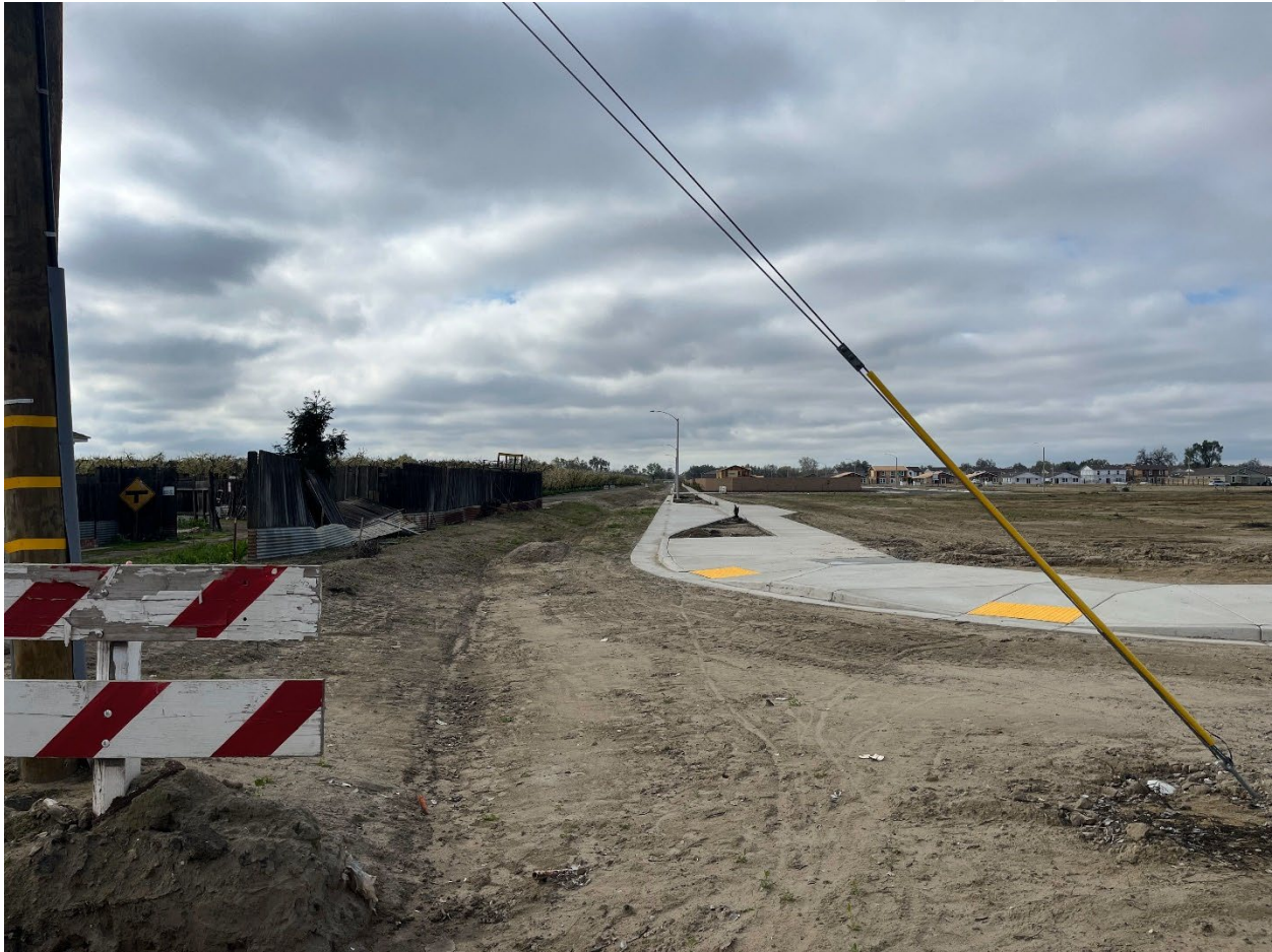
Figure 13— Overview from northwest corner of Project area, facing south
