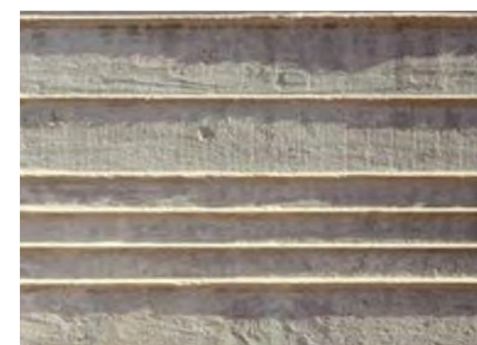
Articulated Extruded Joints
