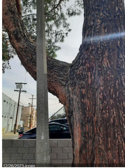
Main scaffold attached at 90° angle.
