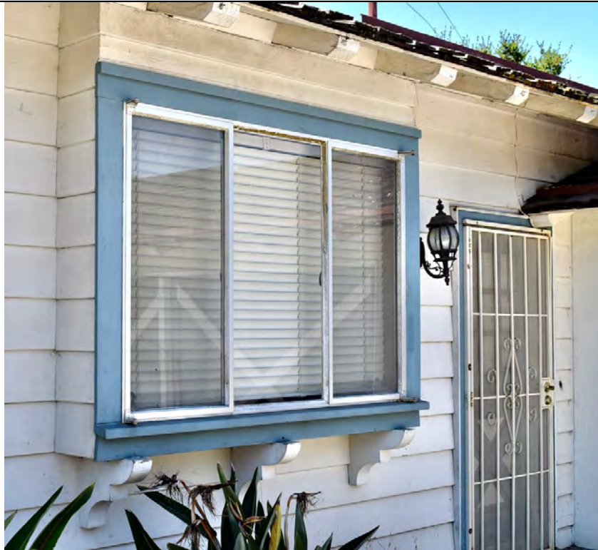
Box oriel window on north façade of main wing
