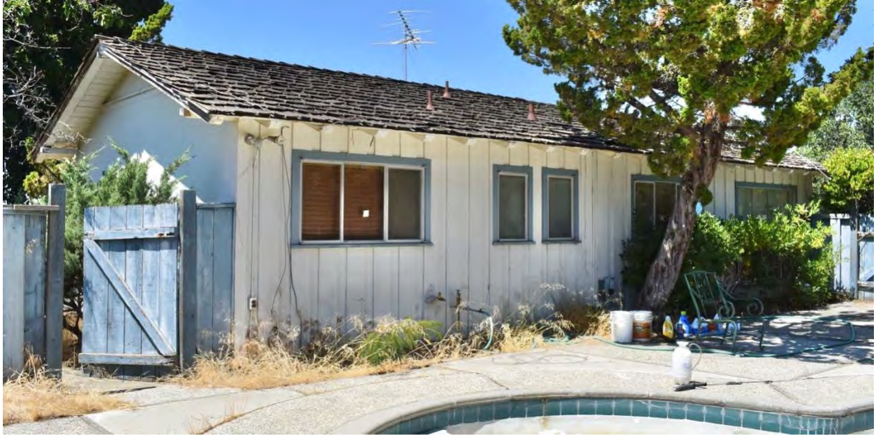
Figure 21: East façade of east wing
