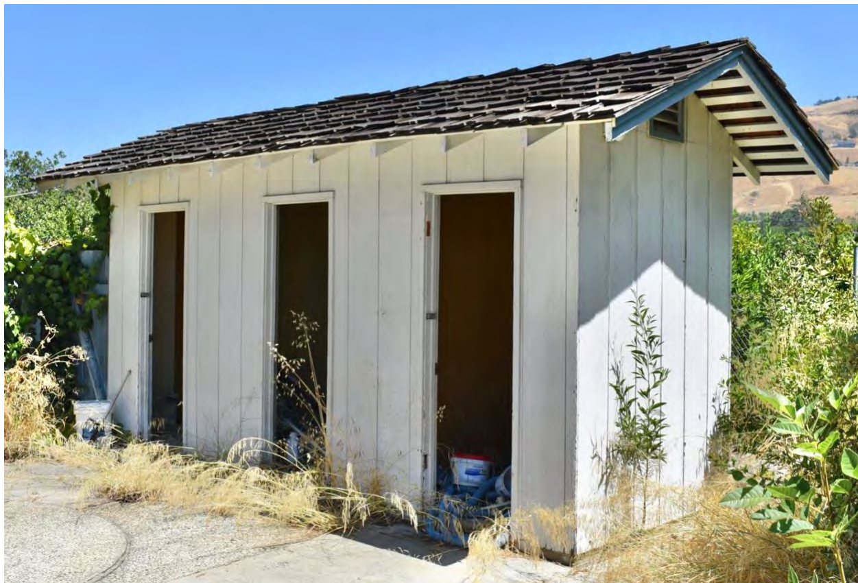
Figure 34: Pool and pool house looking east (top left); mechanical equipment at back of pool house (top left); west and south sides of pool house (bottom)
