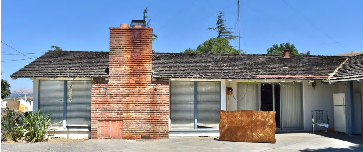
South façade of western part of main wing, with den chimney
