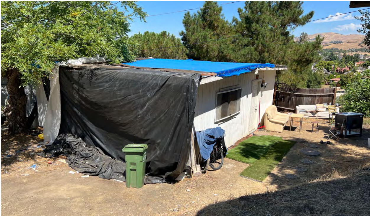
Large storage shed
