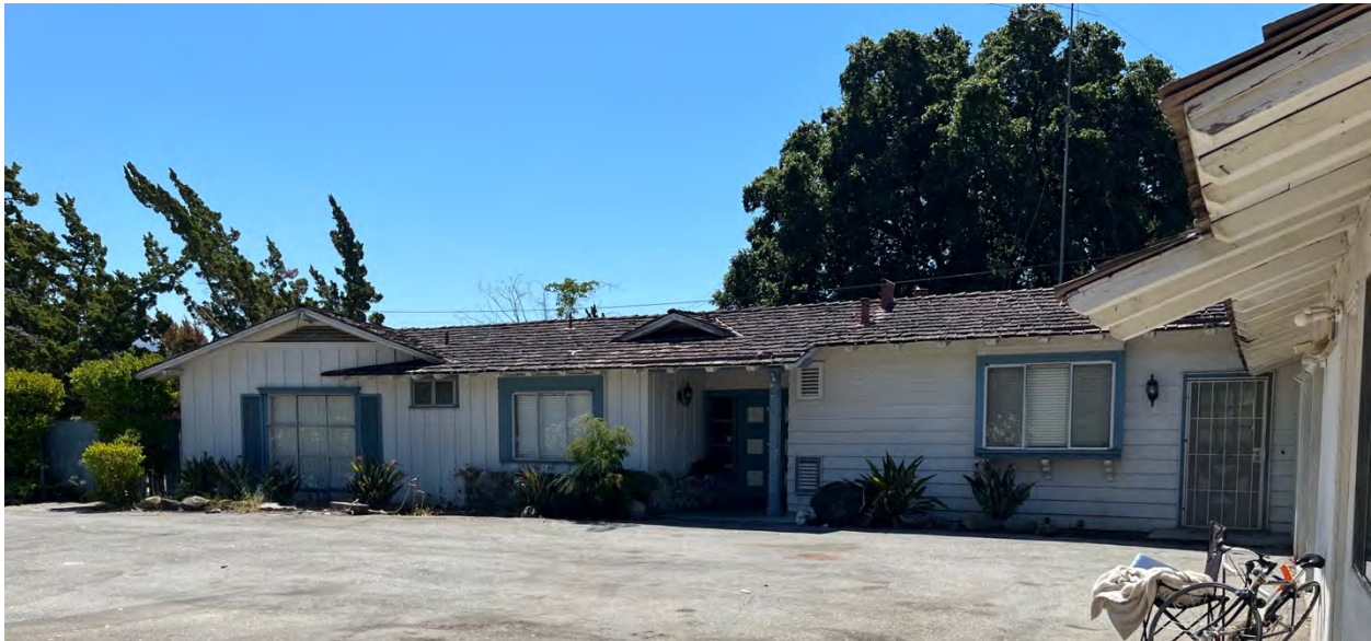
North façade of main and east wings
