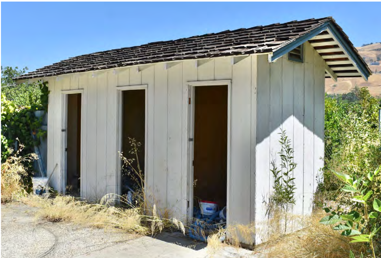
Pool and pool house looking east (top left); mechanical equipment at back of pool house (top left); west and south sides of pool house (bottom)
