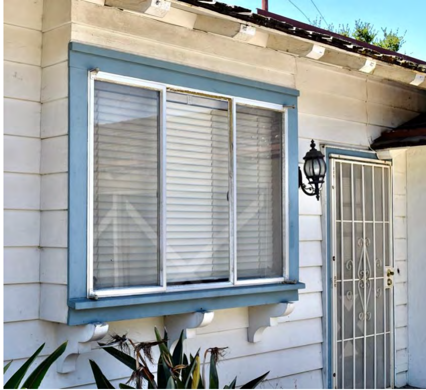
Figure 25: Box oriel window on north façade of main wing
