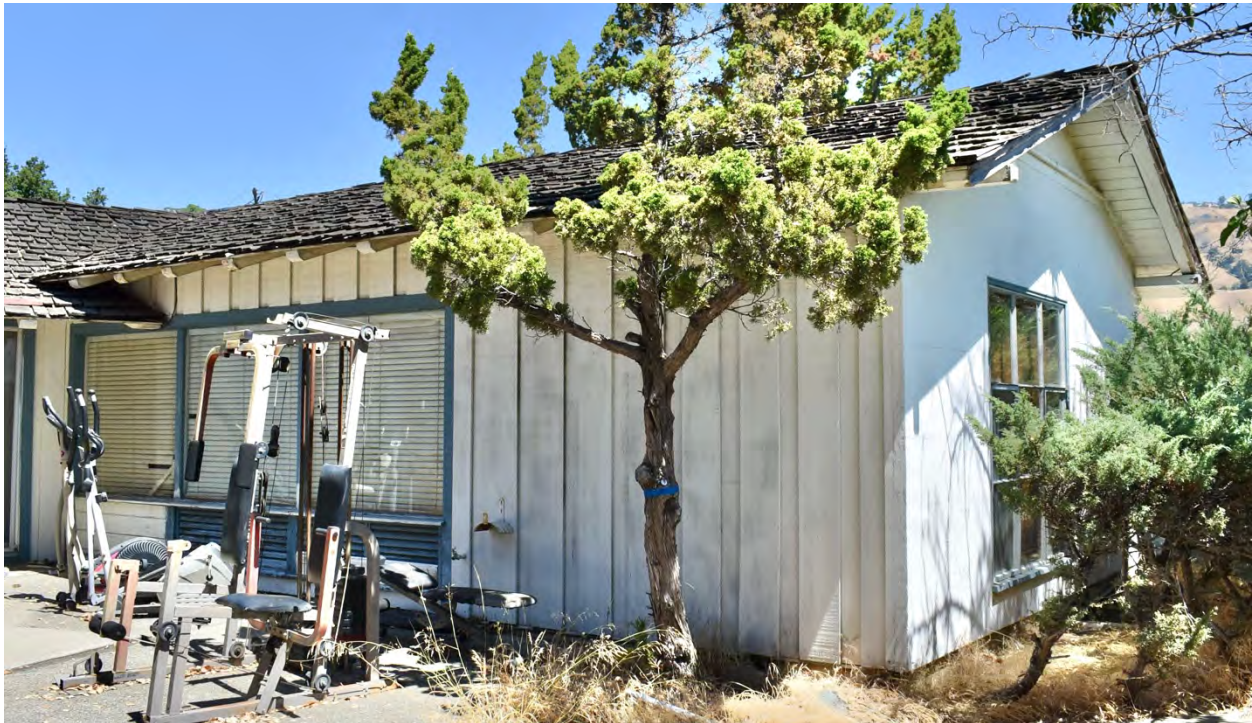
West and south façades of east wing
