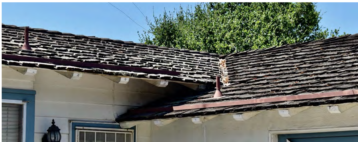
Roof detail at intersection of main and north wings
