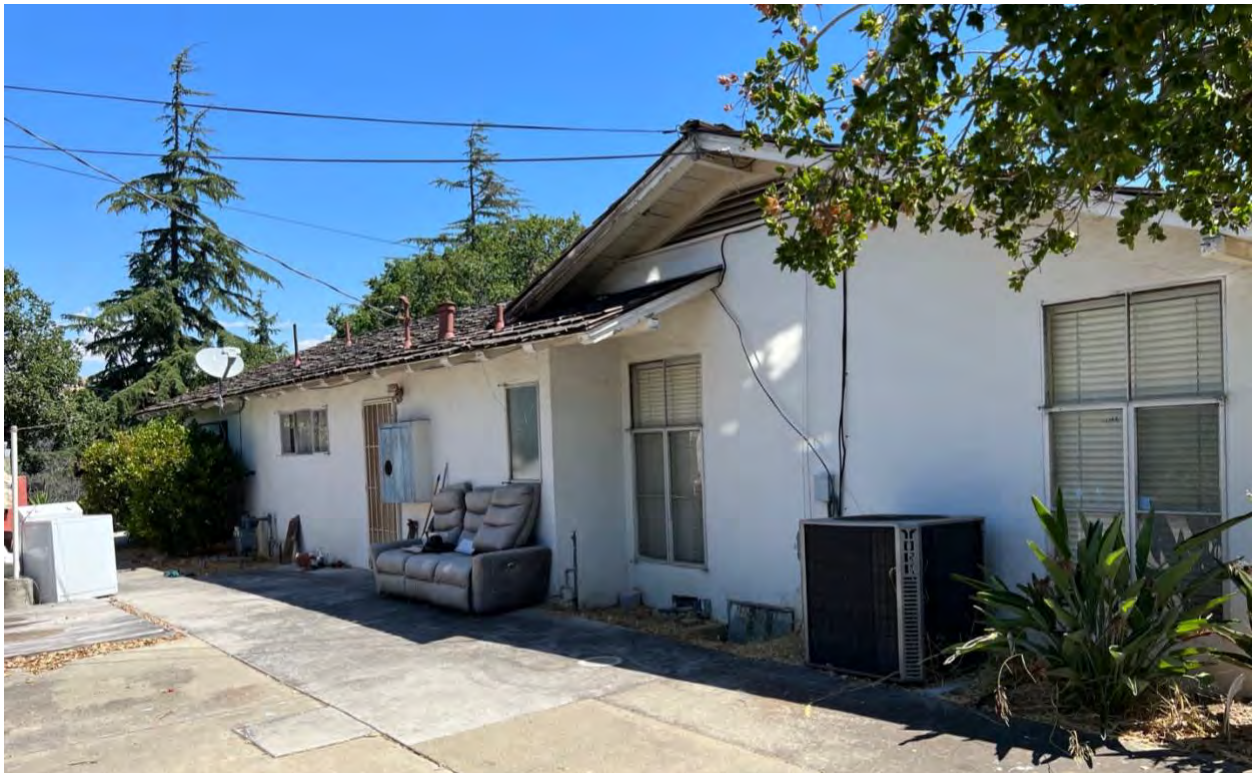
Figure 16: West façade of north wing
