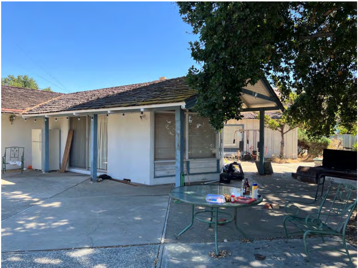
Figure 18: West and south façades of south wing
