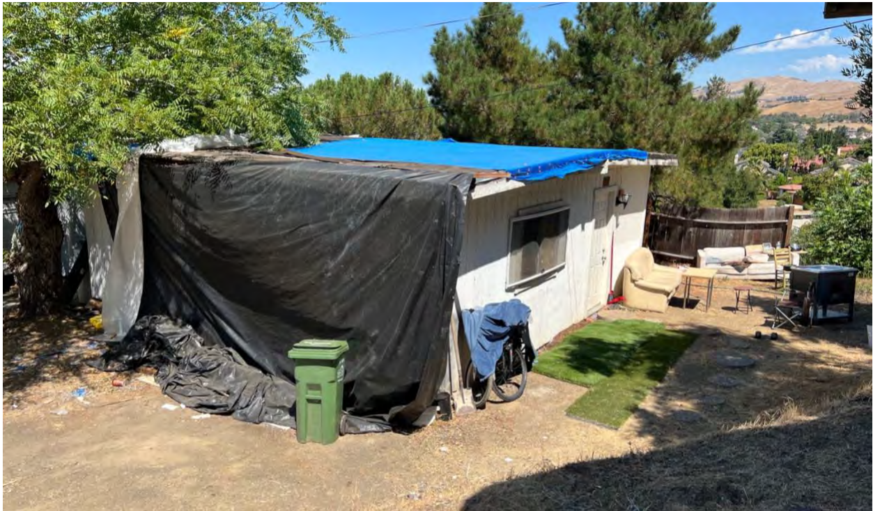
Figure 37: Large storage shed
