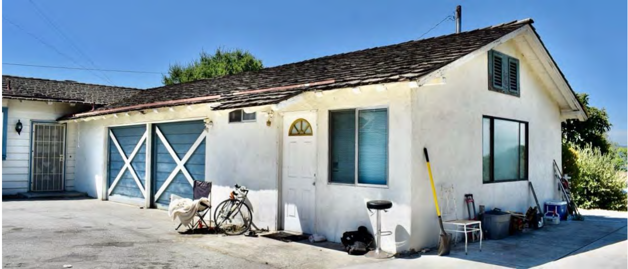
Figure 15: East and north façades of east wing
