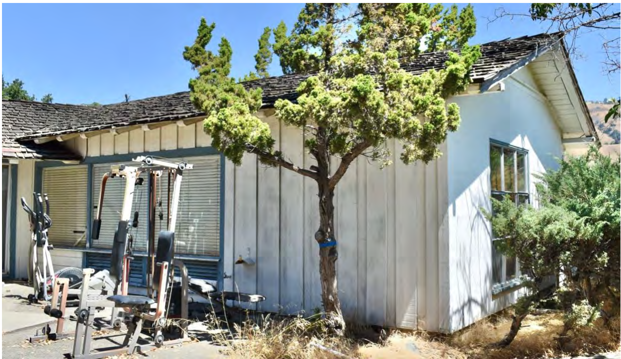
Figure 20: West and south façades of east wing
