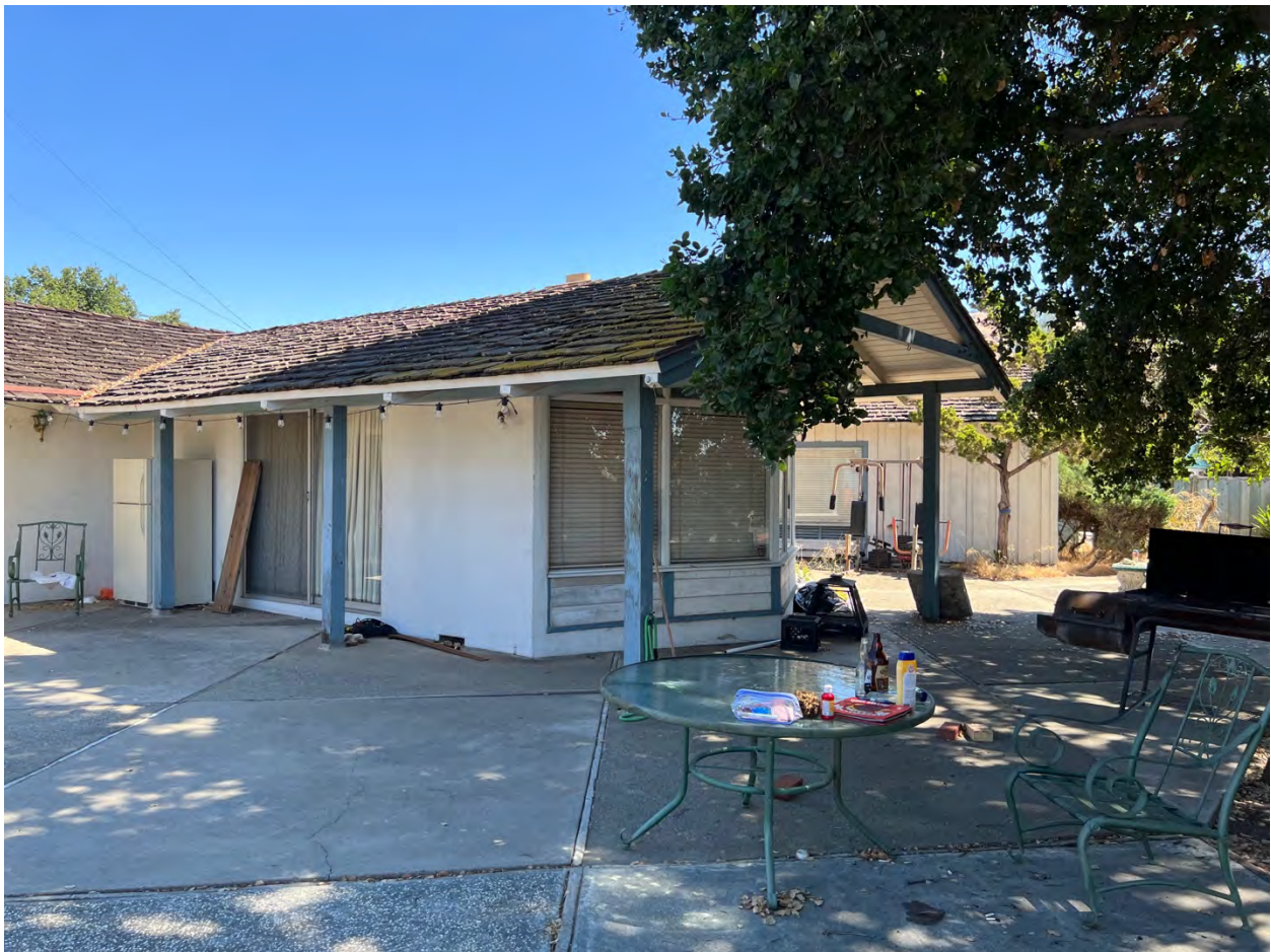
West and south façades of south wing
