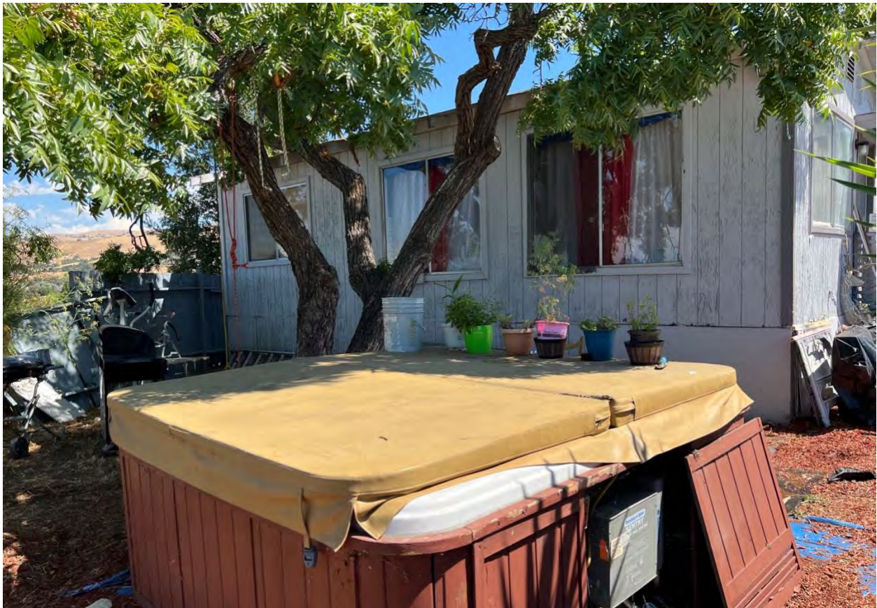
Figure 36: West side of manufactured home
