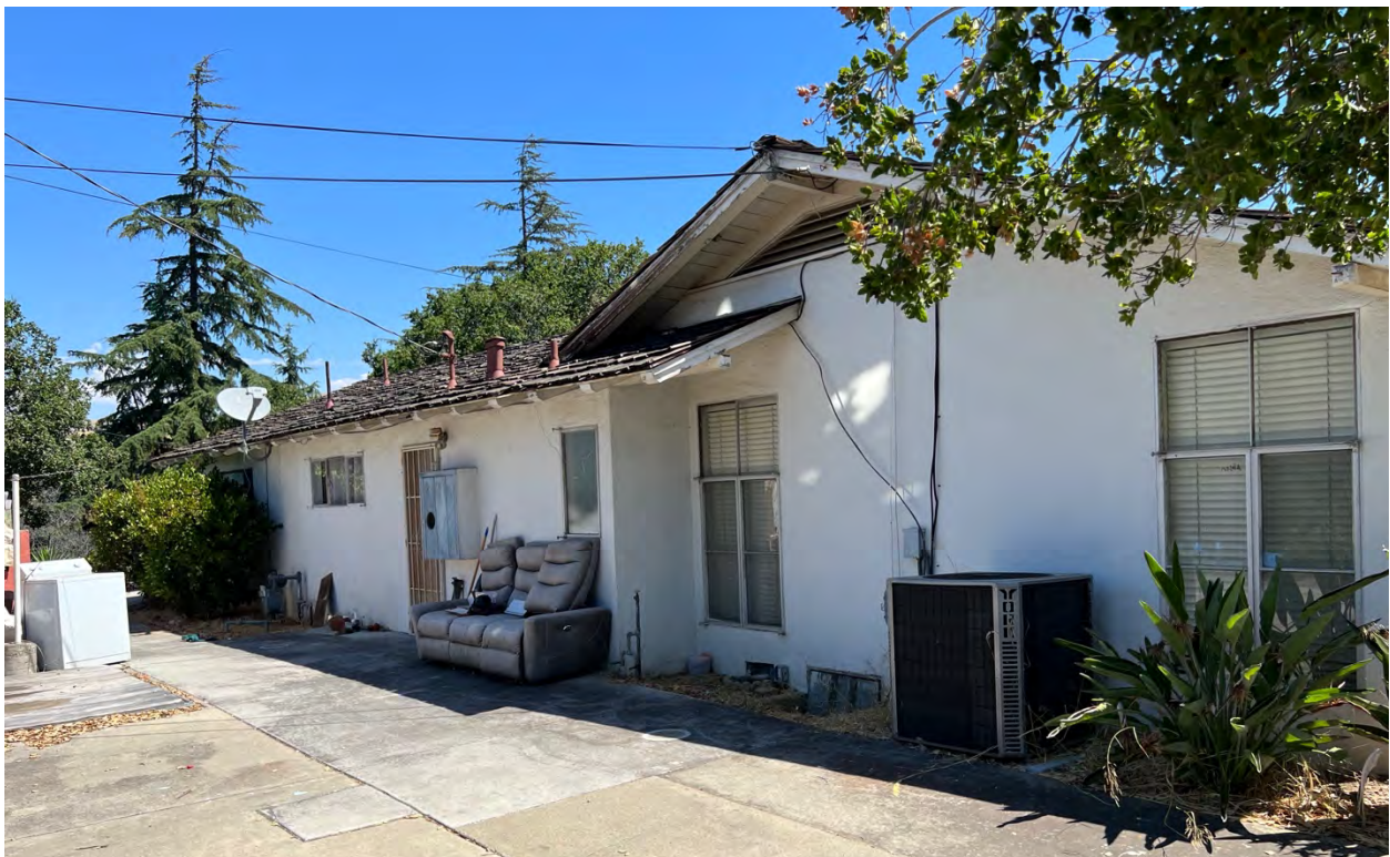
West façade of north wing
