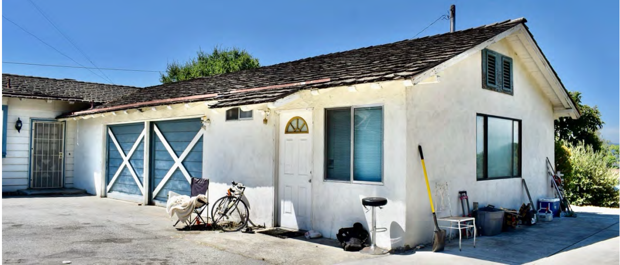
East and north façades of east wing
