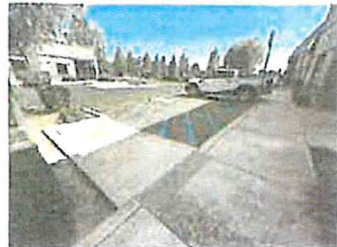
ACCESSIBLE CURB RAMP
