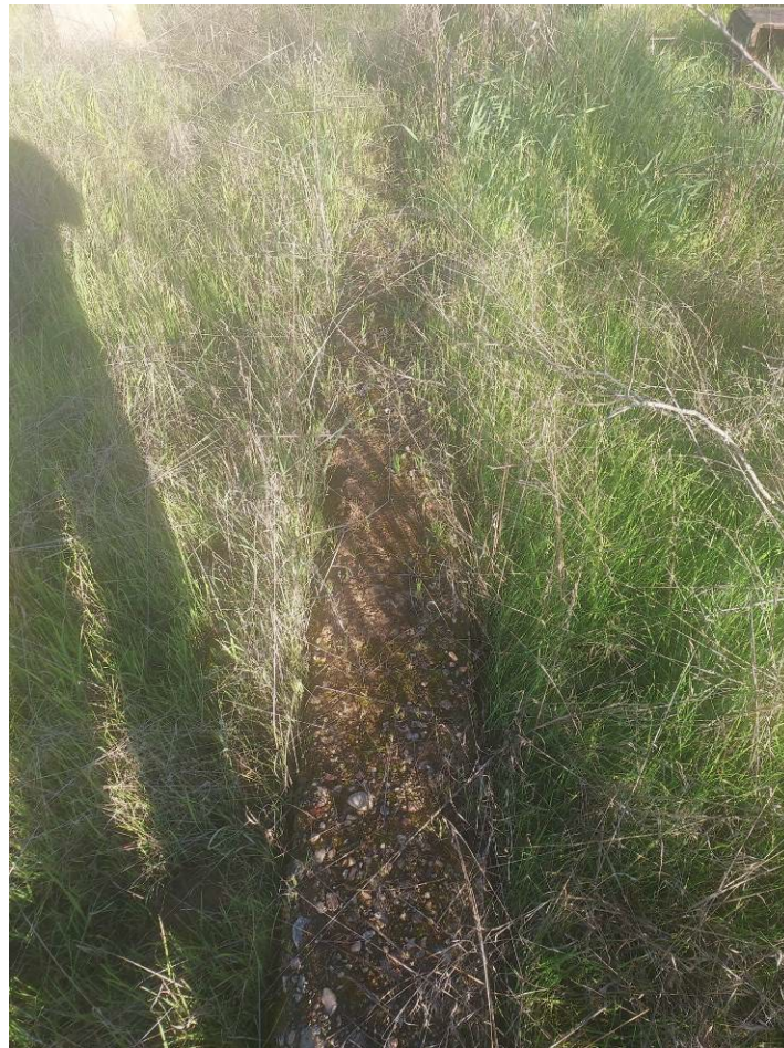
Figure 4 Site C&B-2, Aggregate Concrete Foundation, View to the South
