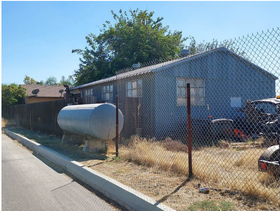
Figure 5 Project Area, Site S-7, Work Building along Sablewood Drive, View to the South
