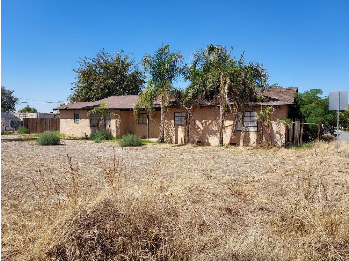
Figure 7 Project Area, Site S-7, House #2, View to the North
