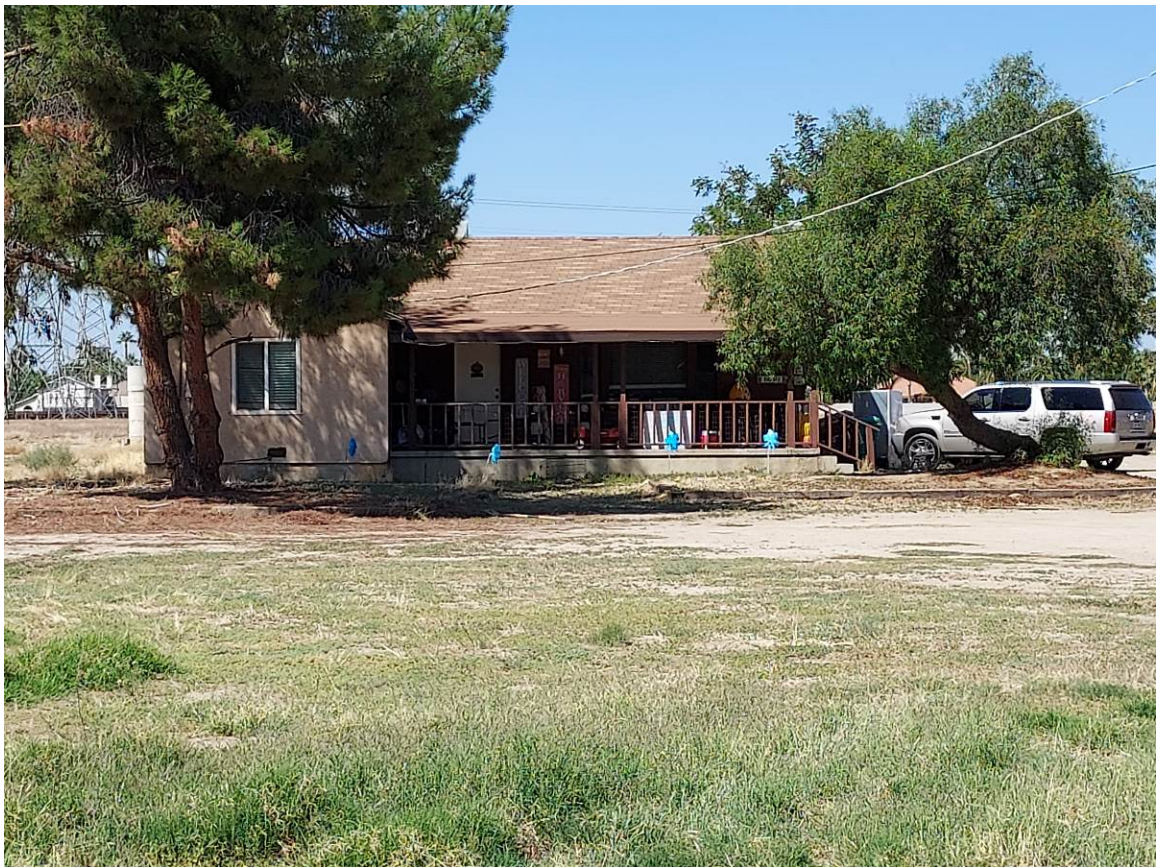
Figure 3 Project Area, Site S-7, House #1, View to the North
