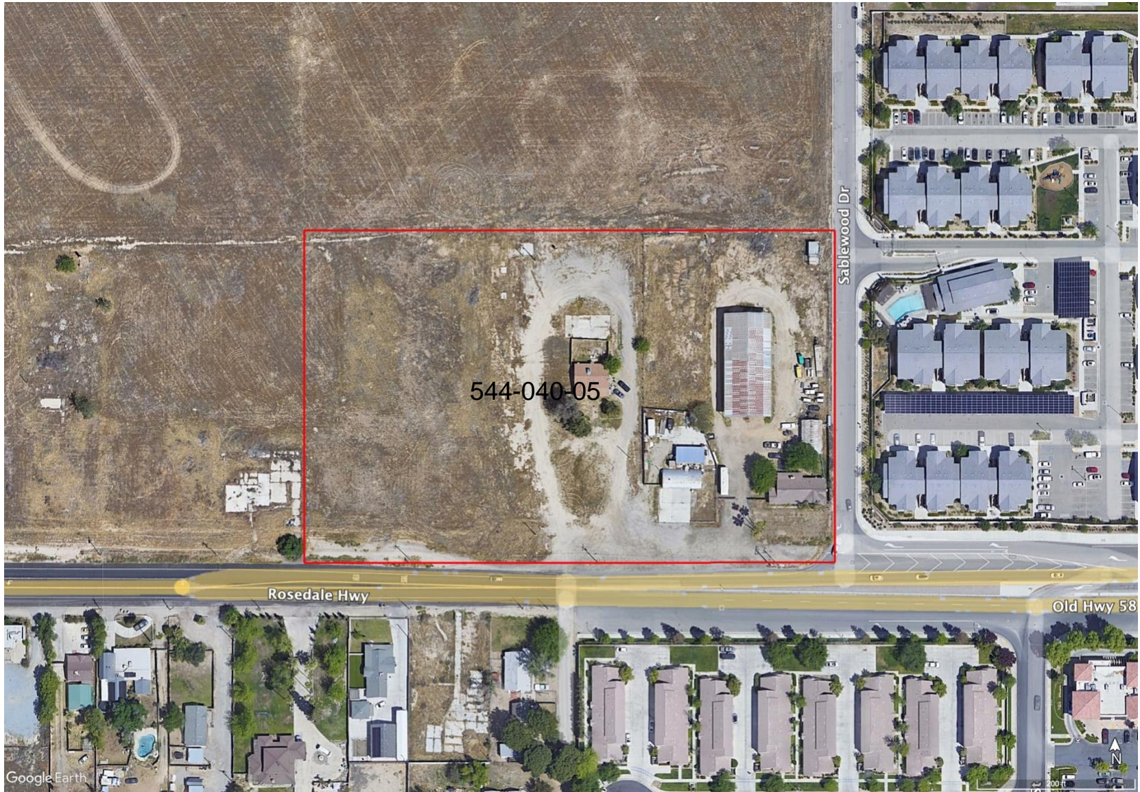
Figure A-2. Aerial photograph of the project and vicinity (Google Earth Pro 2023).
