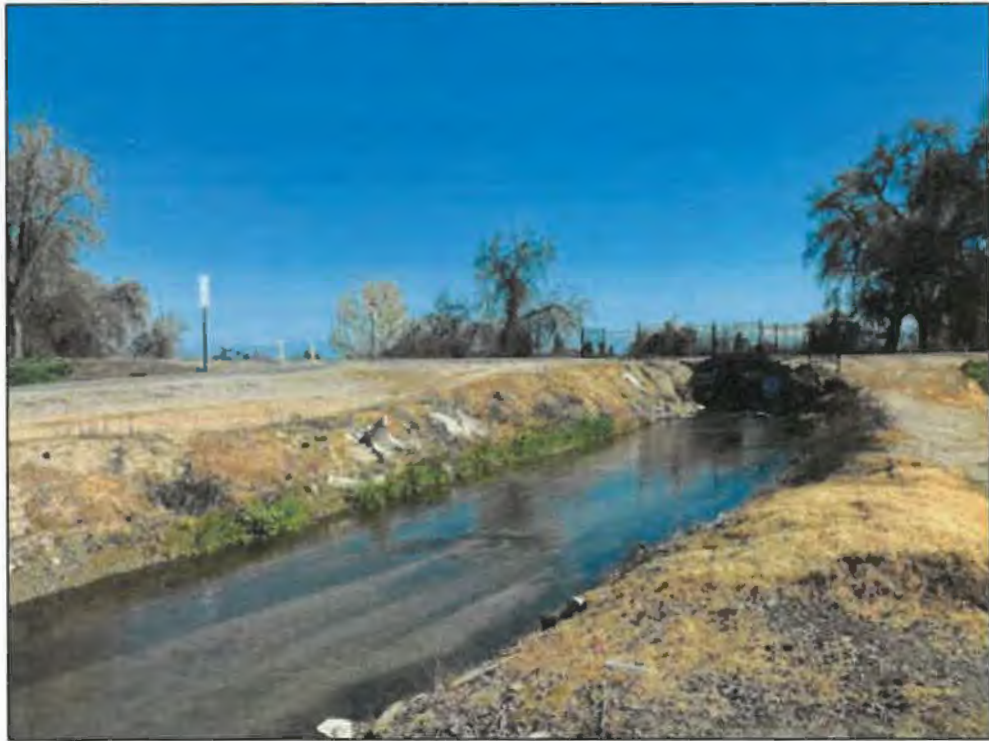
Figure 8. Modoc Ditch, view toward northeast.
