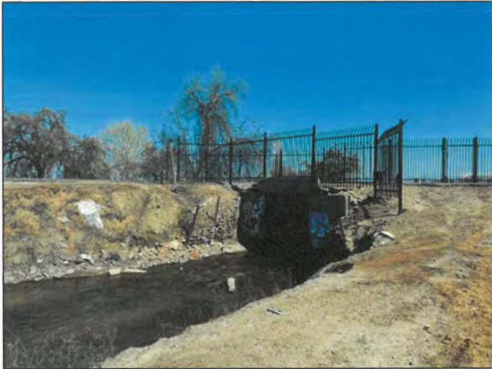
Figure 11. Modoc Ditch headgate outlet structure (culvert), view toward northeast.
