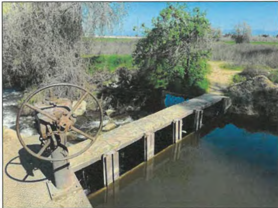
Figure 9. Modoc Ditch checkgate. View toward northeast.
