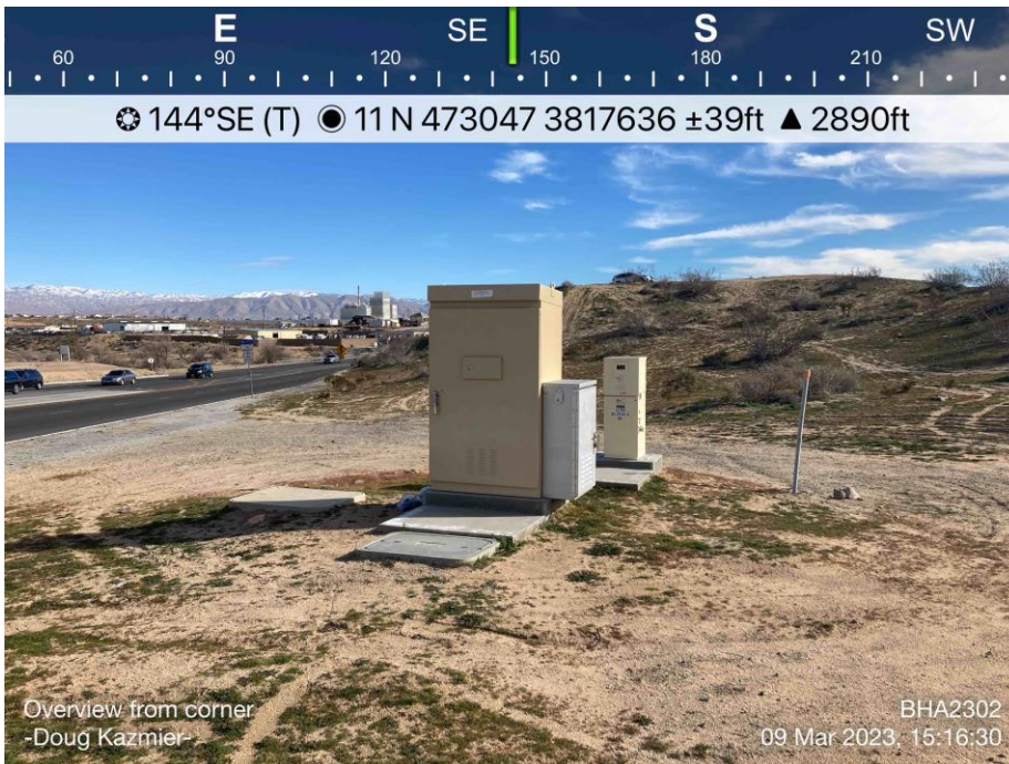
Photo 2: Overview from NE corner (View SSE)
