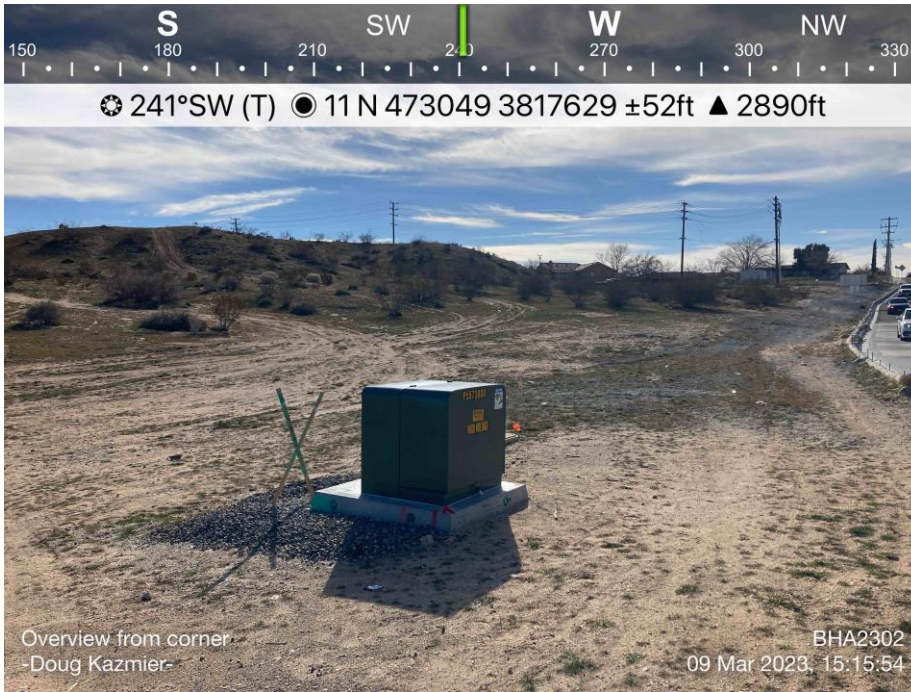
Photo 1: Overview from NE corner (View WSW)
