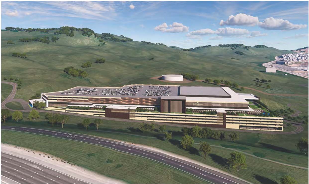
SCOTTS VALLEY RESORT | Exterior View 04
