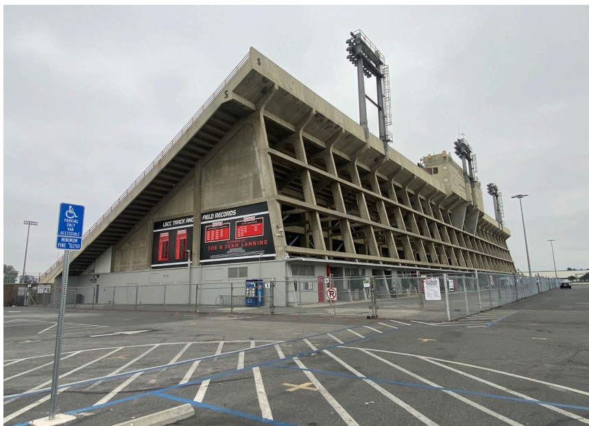
Veterans Memorial Stadium, north and west elevations, facing southeast
