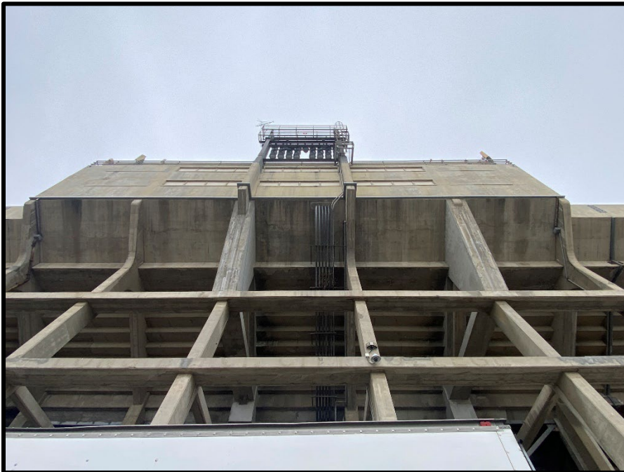
Veterans Memorial Stadium, west elevation, reinforced concrete addition detail
