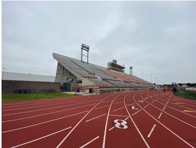
Veterans Memorial Stadium, south and east elevations, facing northwest
