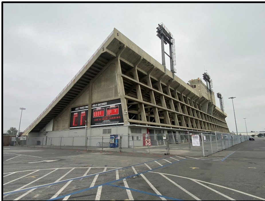
Veterans Memorial Stadium, north and west elevations, facing southeast
