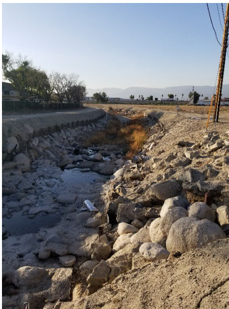
Photograph 1. Looking Northwest at Mission Zanja Channel. Note soft bottom and sides with rip rap are currently in place for stabilization.
