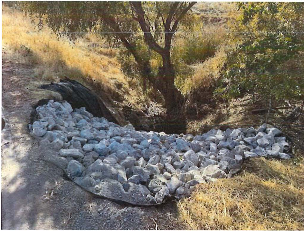
Photo 3. Temporary Winterization Repair at Culvert Inlet
