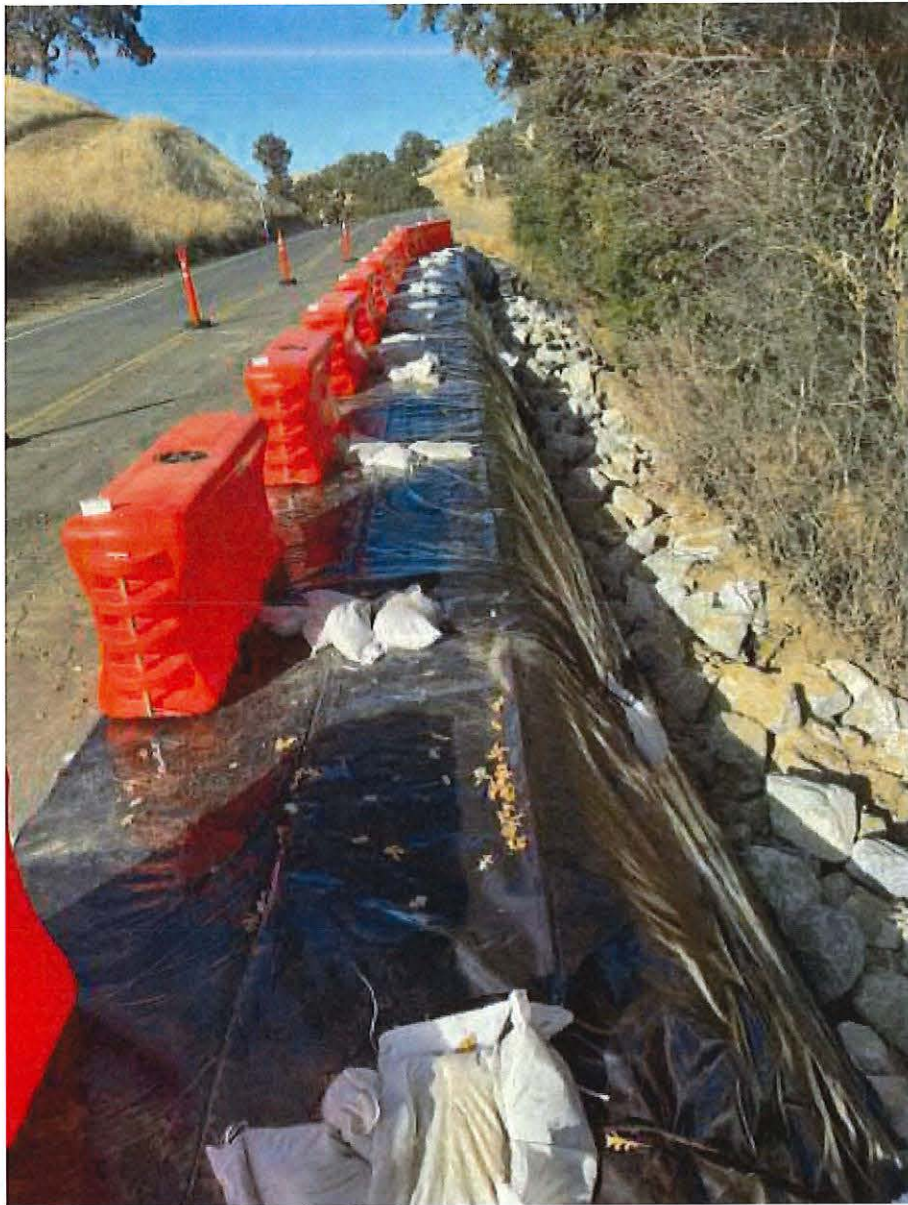
Photo 4. Temporary Winterization Repair at NB Lane
