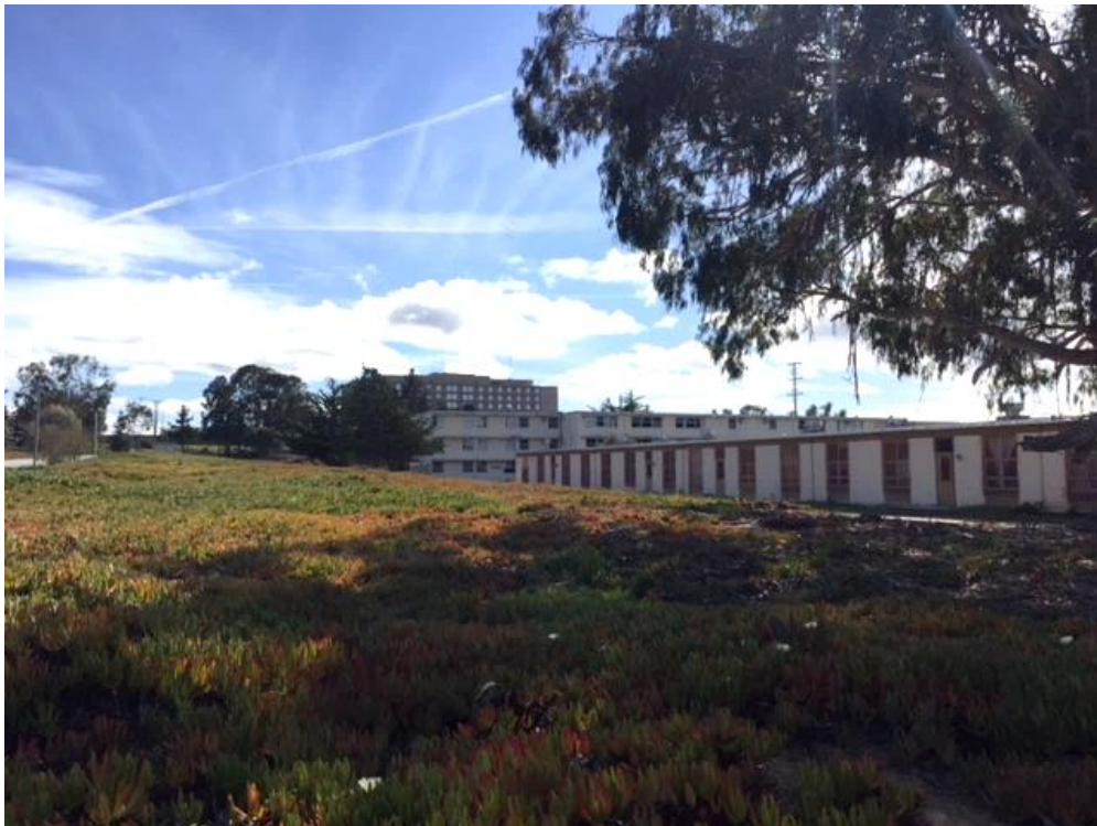
Photograph 14. Existing buildings in Plan Area, looking south on Colonel Durham Street near 6 th Avenue
