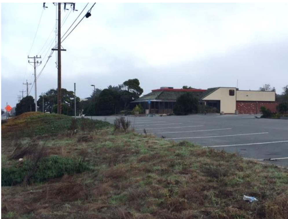
Photograph 4. Abandoned commercial building and parking lot, looking northeast from the intersection of General Jim Moore Boulevard and Gigling Road
