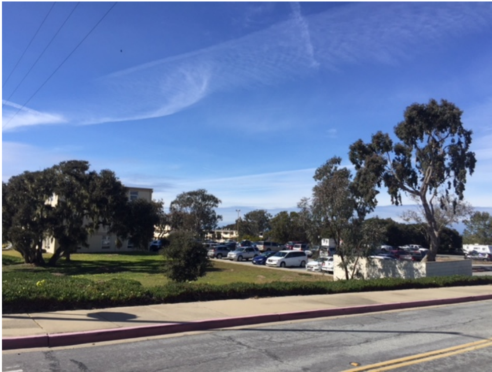
Photograph 9. Existing buildings south of Plan Area, looking northwest along Parker Flats Road near Gigling Road
