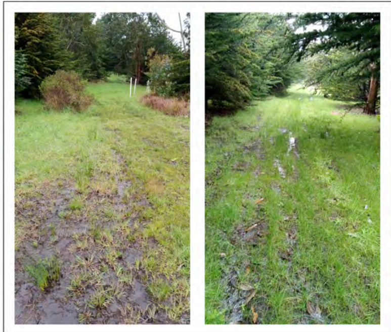
Figure 12: Alternate Access Driveway (titled Grass Path in Figure 1) Within Presumed Wetland ESHA
