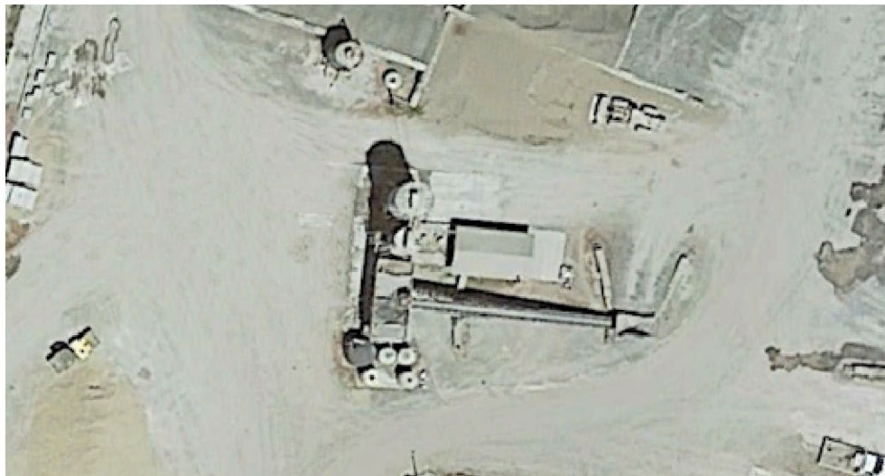
Figure 2 Ready-Mix Batch Plant
