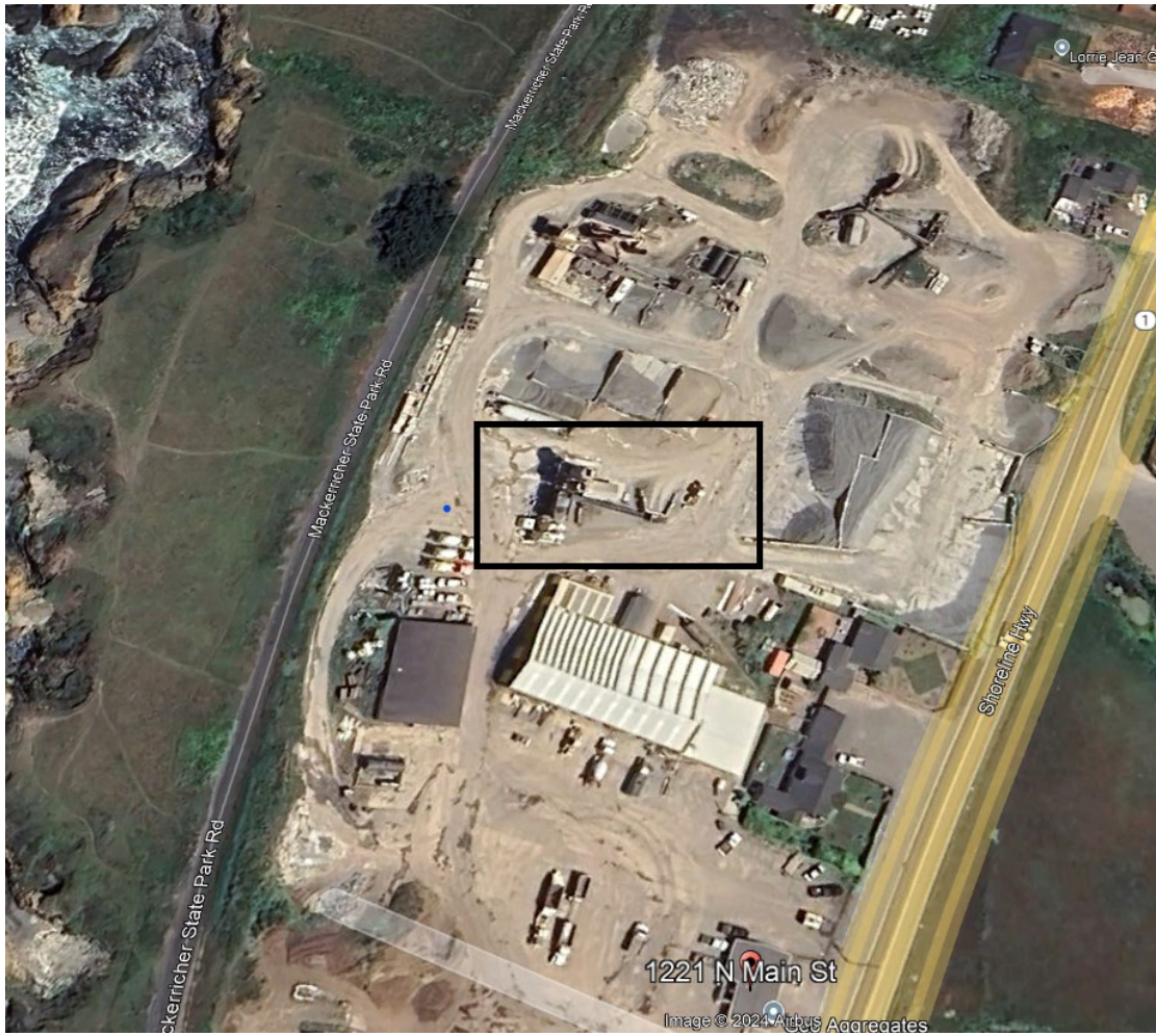
Figure 1 - Aerial View Site; Ready-Mix Batch Plant
