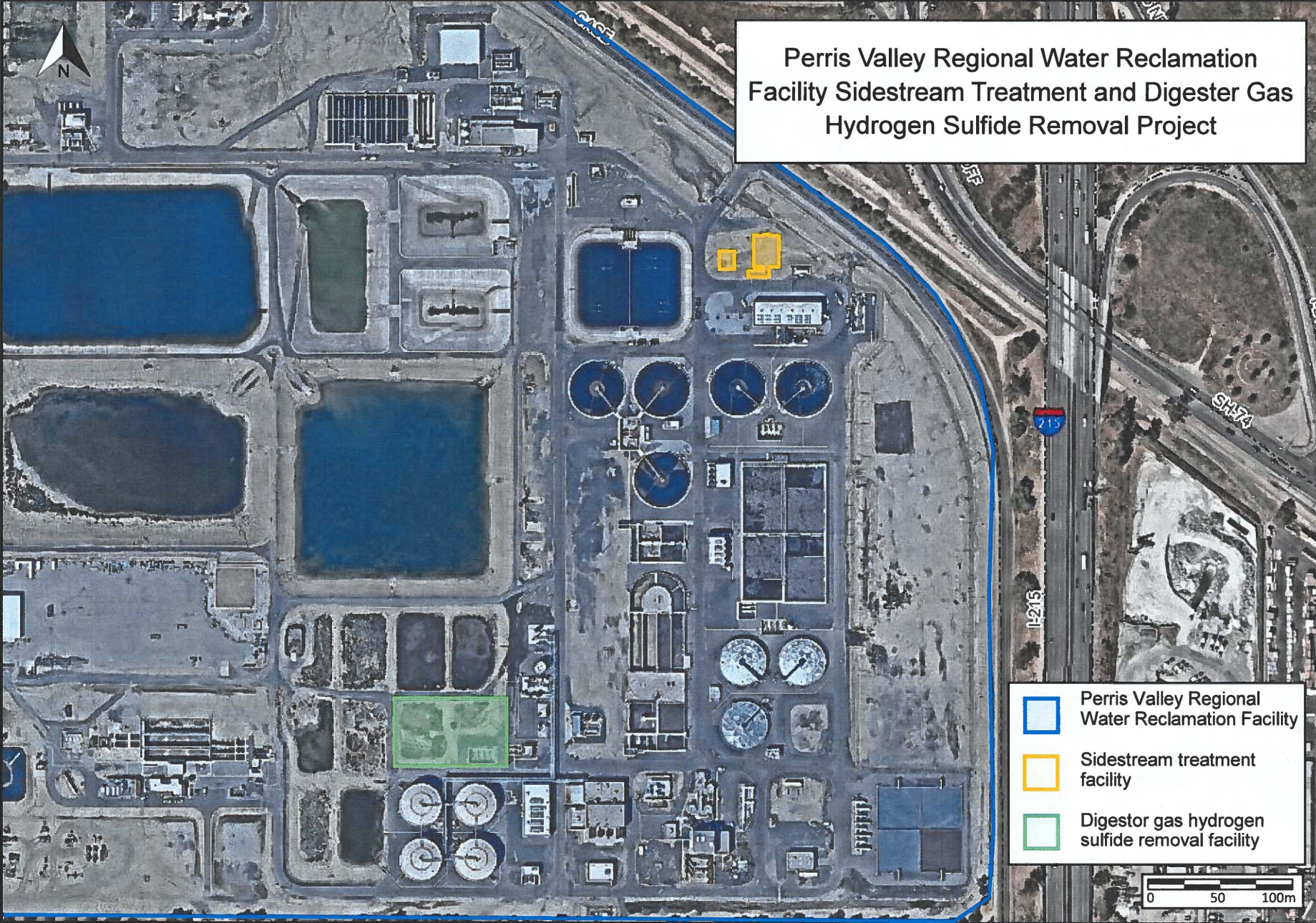
PVRWRF Sidestream Treatment and Digester Gas Hydrogen Sulfide Removal
