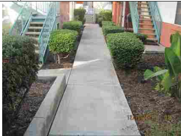
41- Typical Concrete Walkway
