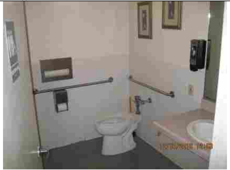
36- Common Building Bathroom
