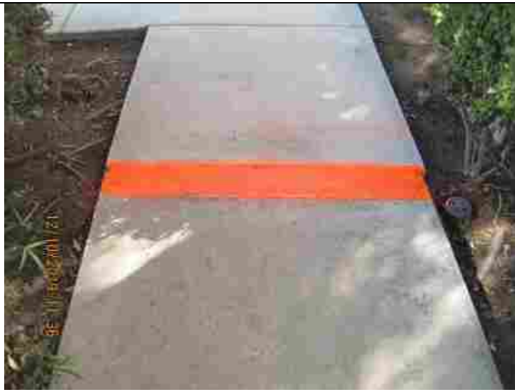
43- Concrete Repairs in Progress
