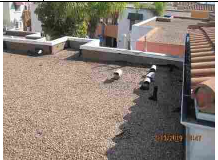
48- Typical Roof Views
