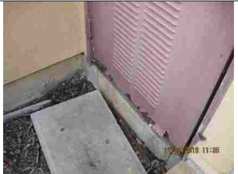
10- Typical Utility Closet Door
