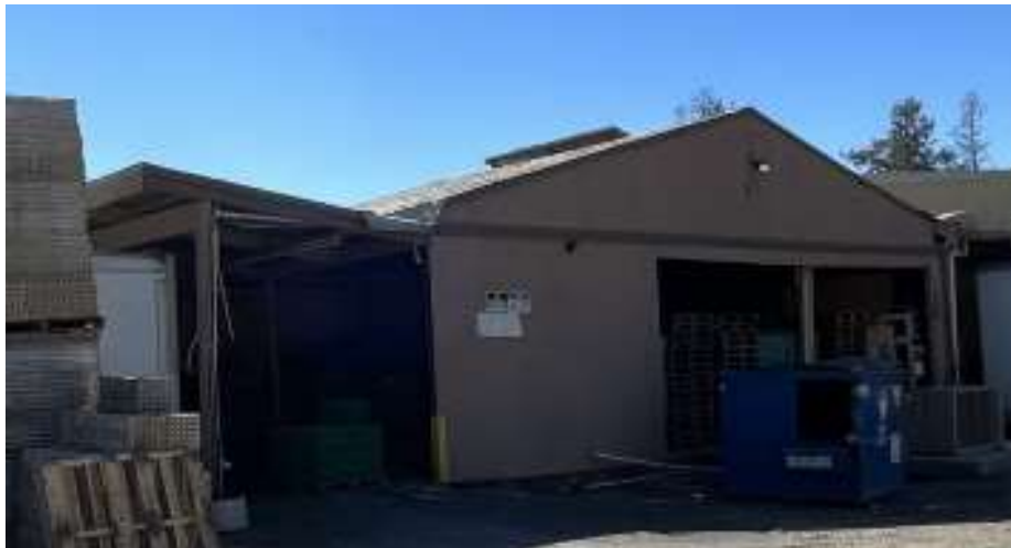
Figure 10. East elevation of Building 2 (August 2022).
