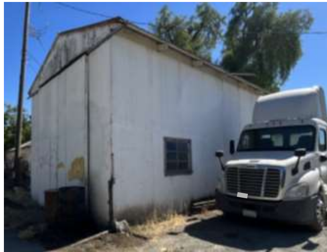
Figure 28. North and east façades of Building 7 (August 2022).
