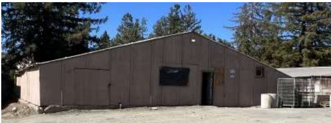
Figure 31. South and west façades of Building 9 (August 2022).
