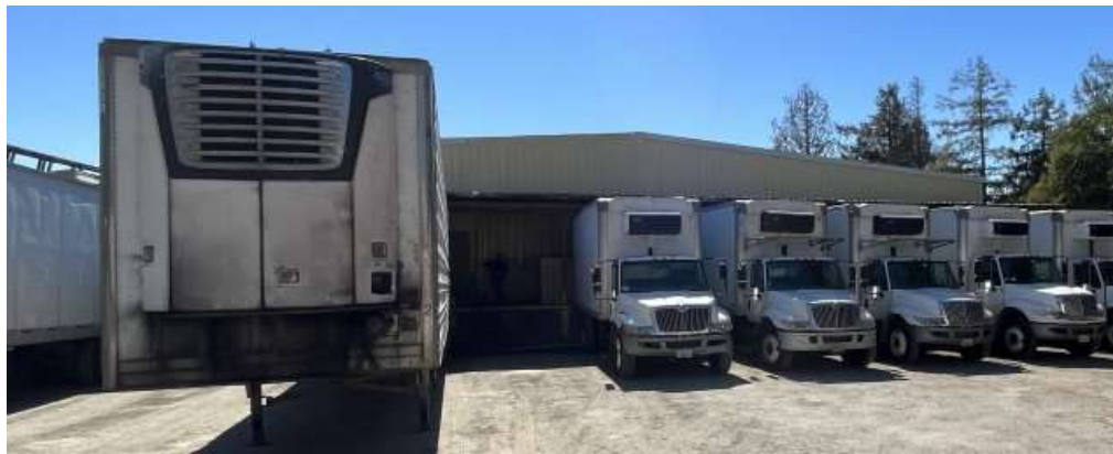
Figure 7. East elevation of Building 1 (August 2022).
