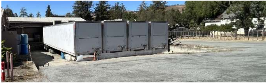
Figure 11. The loading dock, view from Sierra Road (August 2022).
