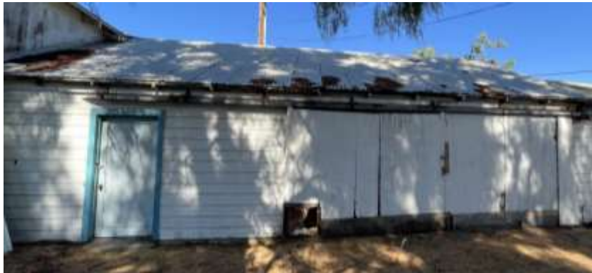
Figure 25. West façade of Building 6 (August 2022).
