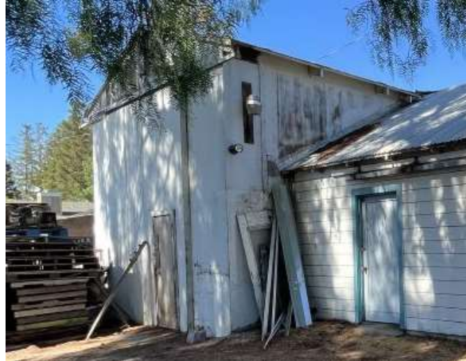
Figure 27. West and south façades of Building 7 (August 2022).
