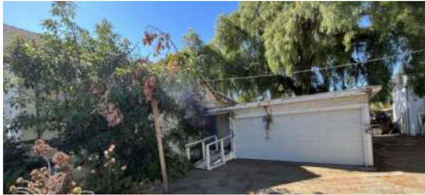
Figure 19. The garage of Building 4 (August 2022).
