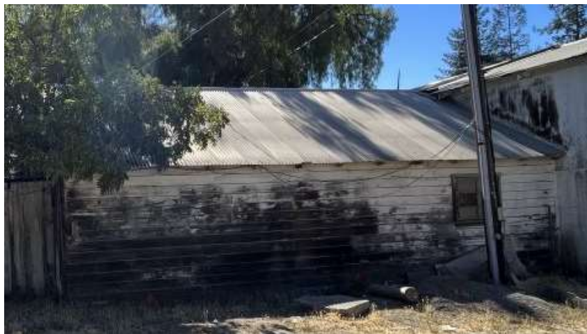
Figure 26. East façade of Building 6 (August 2022).
