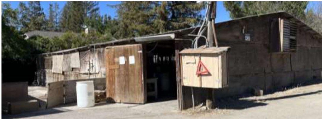
Figure 30. West façade of Building 8 (August 2022).
