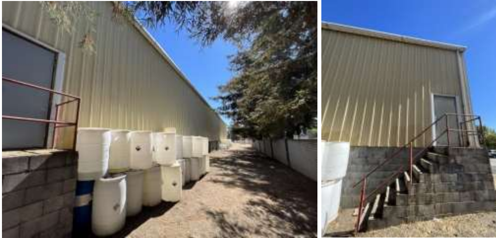
Figures 5 and 6. Details of Building 1's north elevation (August 2022).
