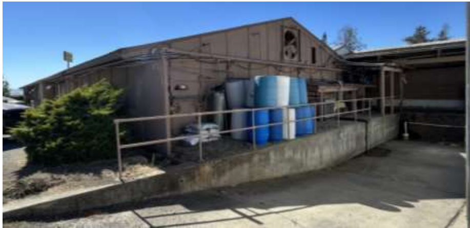
Figure 14. East elevation of Building 3 (August 2022).
