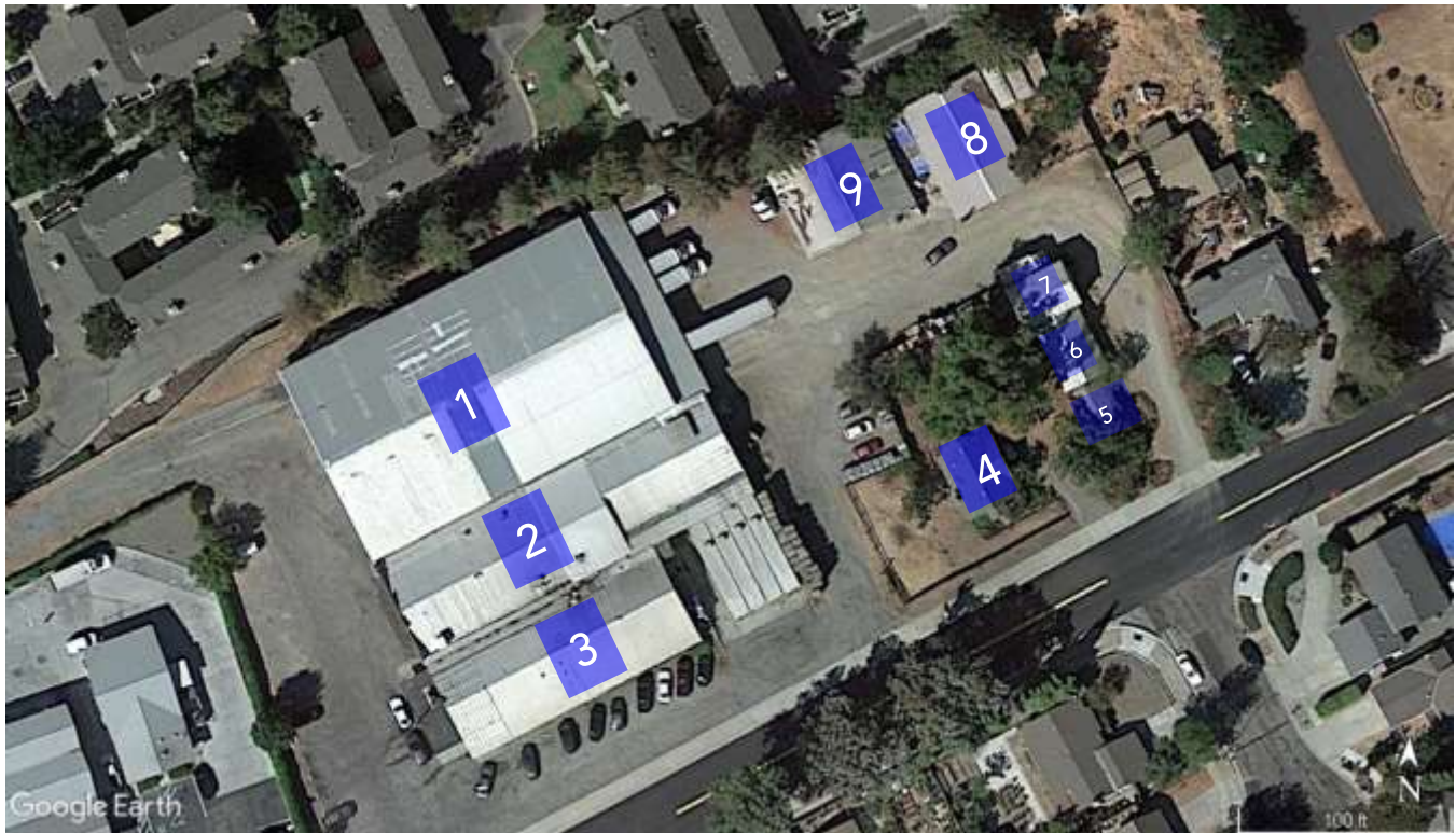
Figure 3. The subject property buildings numbered in blue and white (Google Earth, imagery date September 2021).
