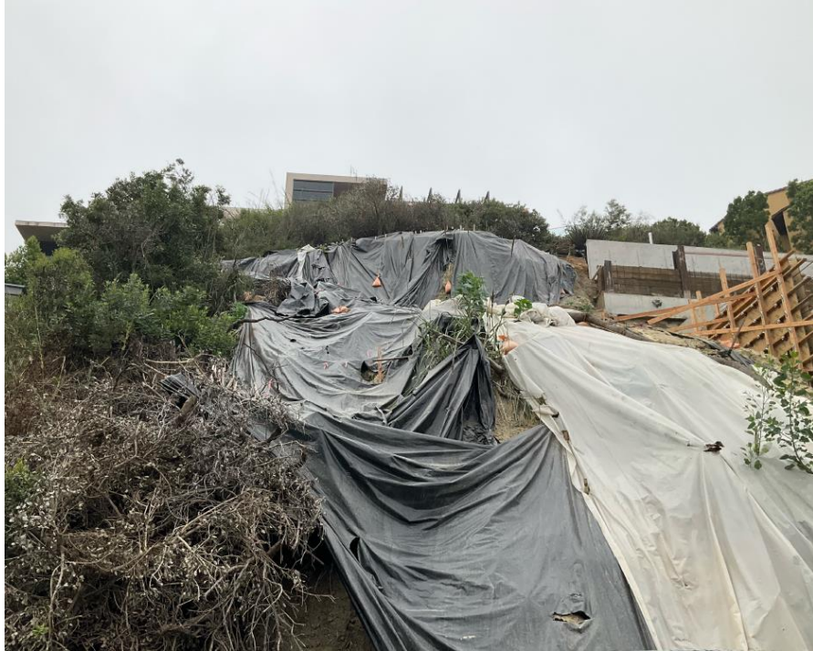
Figure 5-3. View of Project area looking upslope from Gainsborough Drive, facing southeast.
