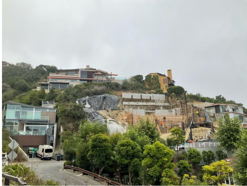
Figure 5-1. Overview of Project area (left) and in-development property (right), facing south.
