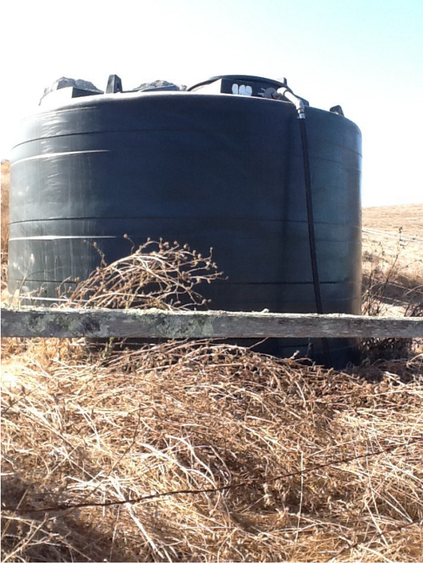
Upper Storage Tank
