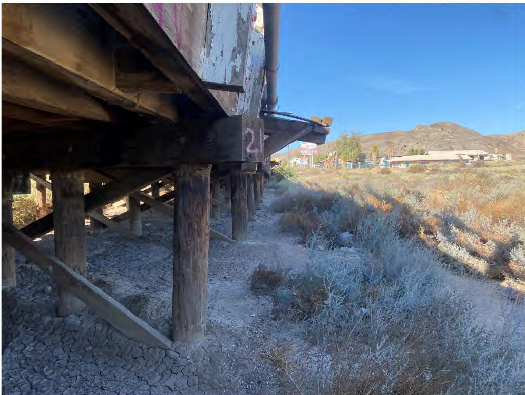
Photo 8. Typical view along existing bridge. View facing southwest.
