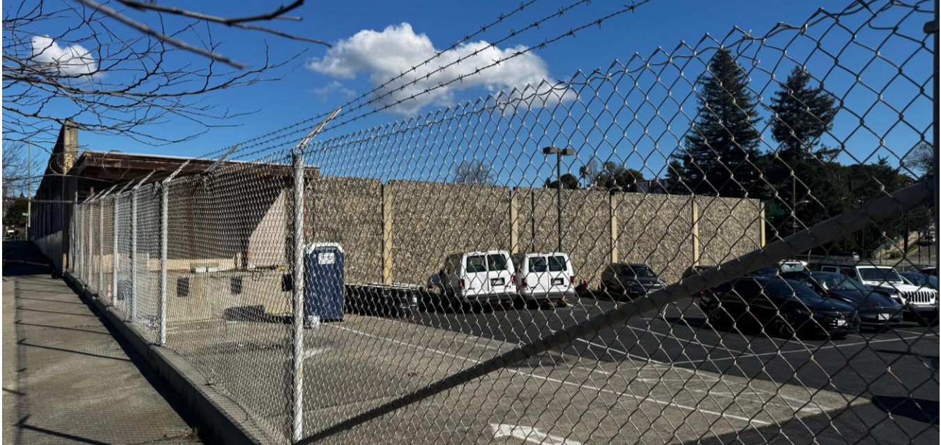
Figure 1. View of the northwest façade. Three façades are pebble walls. Note the loading dock and variation between street and site grade at the left edge of the image. (ESA, 2025)
