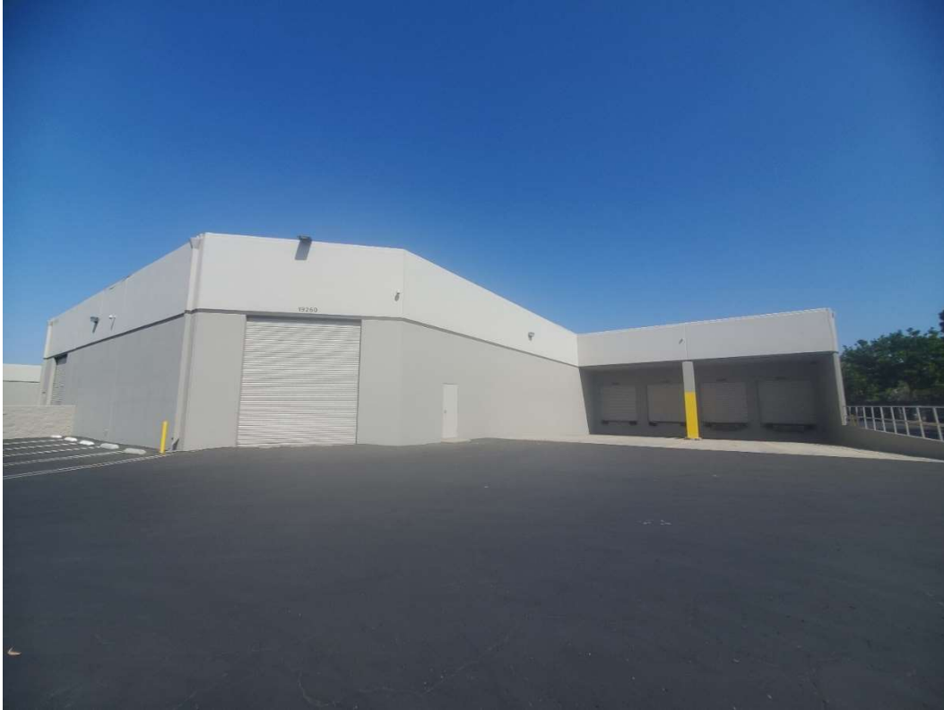
Figure 5-16. 19250 Van Ness Avenue rear (eastern) elevation, facing northwest.
