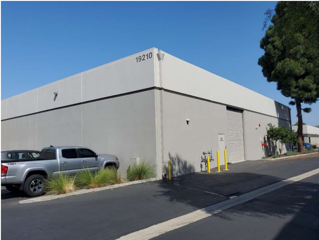
Figure 5-18. 19210 Van Ness Avenue rear (eastern) elevation, facing northwest.
