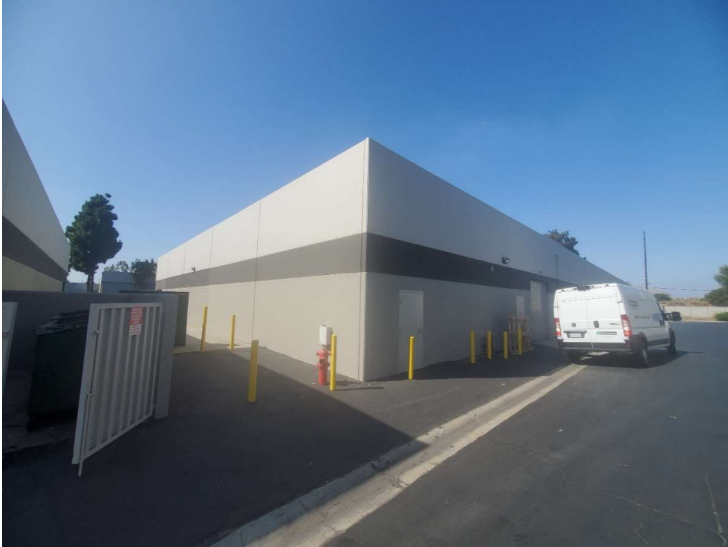
Figure 5-12. 19140 Van Ness Avenue rear (southern) elevation, facing southwest.
