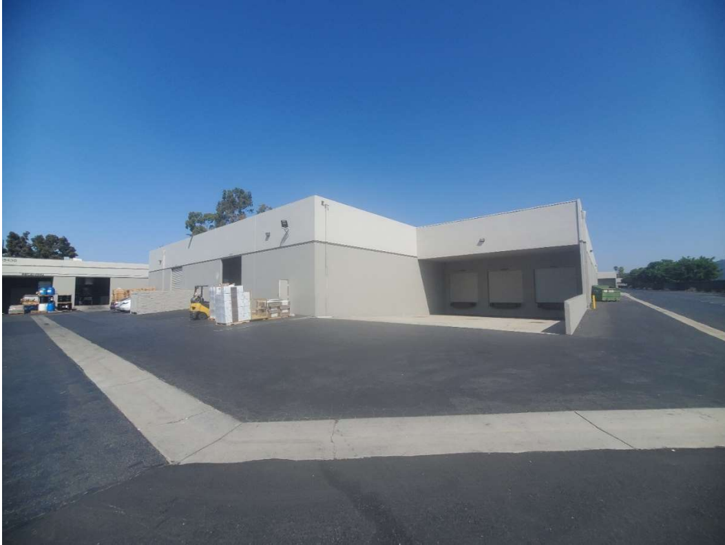
Figure 5-24. 19370 Van Ness Avenue rear (southern) elevation, facing northwest.
