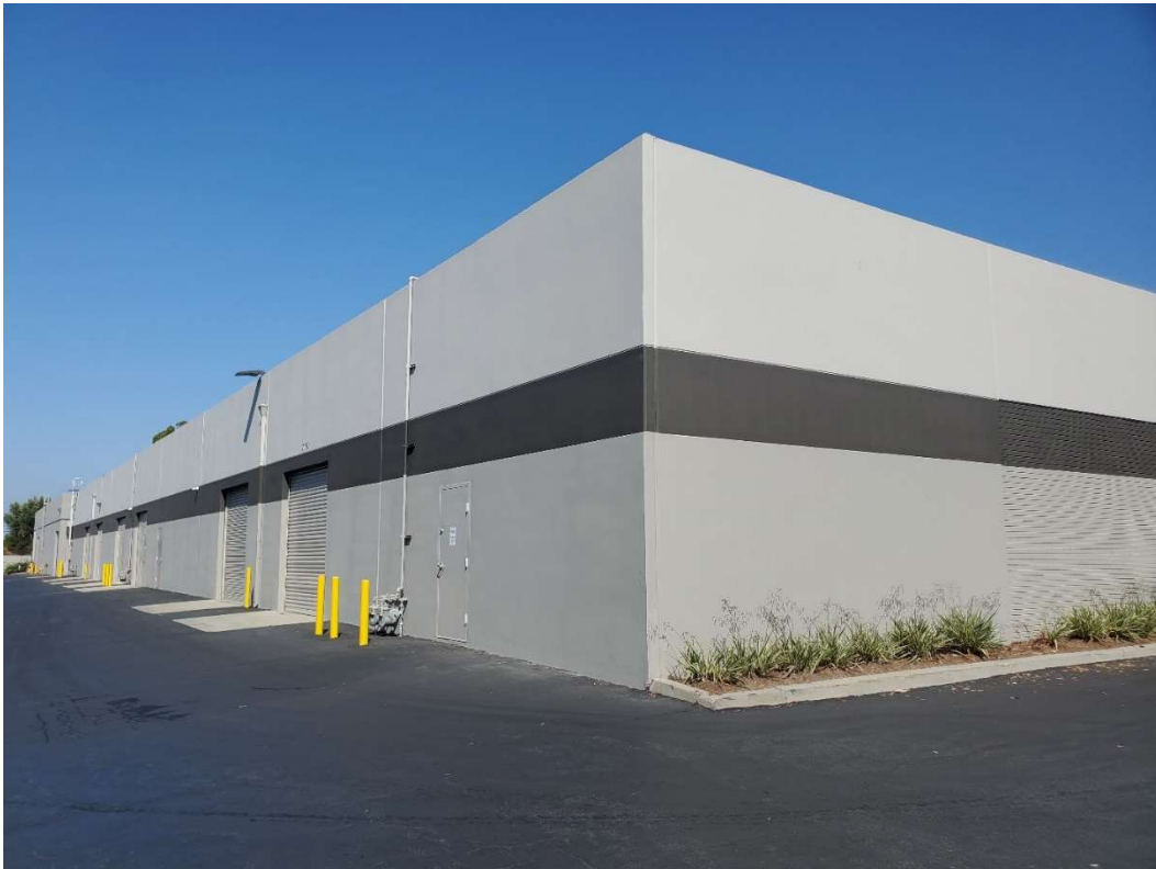
Figure 5-10. 2180 West 190th Street rear (southern) elevation, facing northwest.
