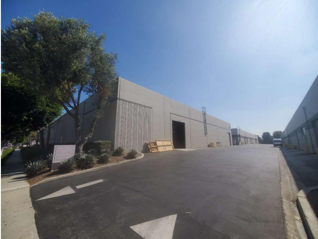
Figure 5-8. 19110 Van Ness Avenue rear (western) elevation, facing northeast.
