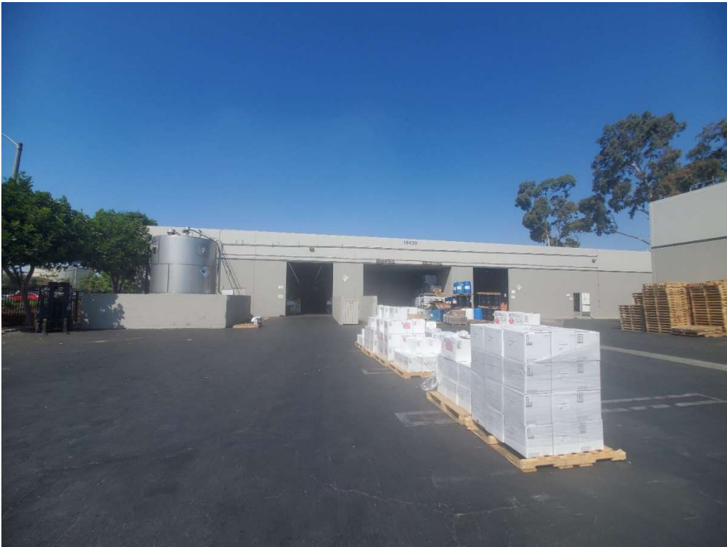
Figure 5-26. 19430 Van Ness Avenue rear (eastern) elevation, facing west.
