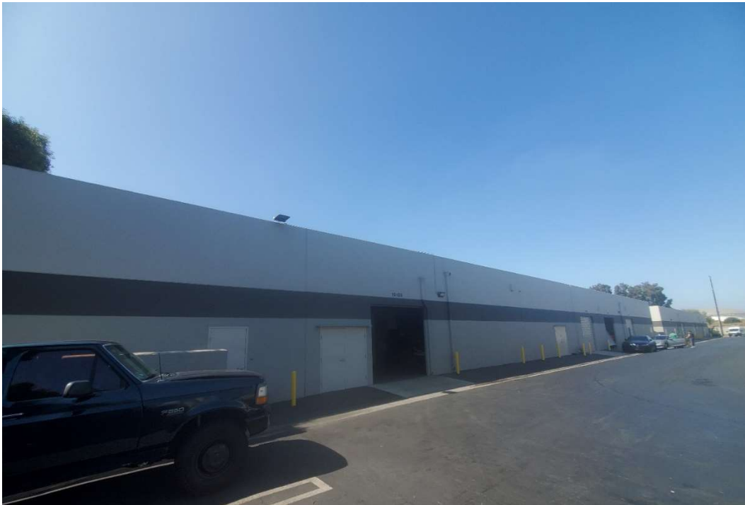
Figure 5-14. 19160 Van Ness Avenue rear (northern) elevation, facing southwest.
