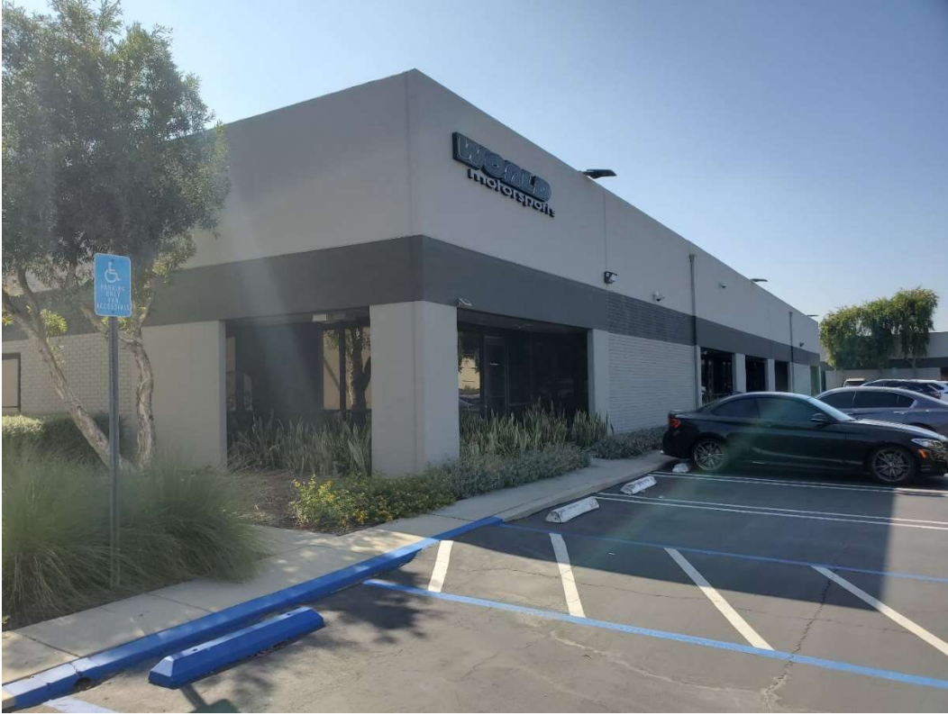
Figure 5-5. 2170 West 190th Street primary (western) elevation, facing southeast.
