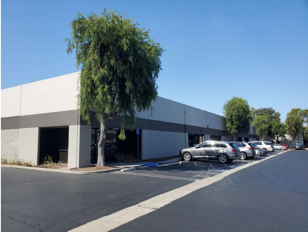
Figure 5-9. 2180 West 190th Street primary (northern) elevation, facing southwest.
