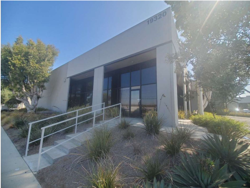
Figure 5-21. 19320 Van Ness Avenue primary (western) elevation, facing east.
