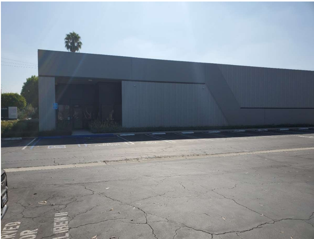
Figure 5-3. 2140 West 190th Street primary (eastern) elevation, facing west.
