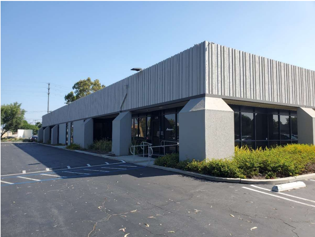
Figure 5-2. Southwestern corner of 2150 West 190th Street, facing northeast.
