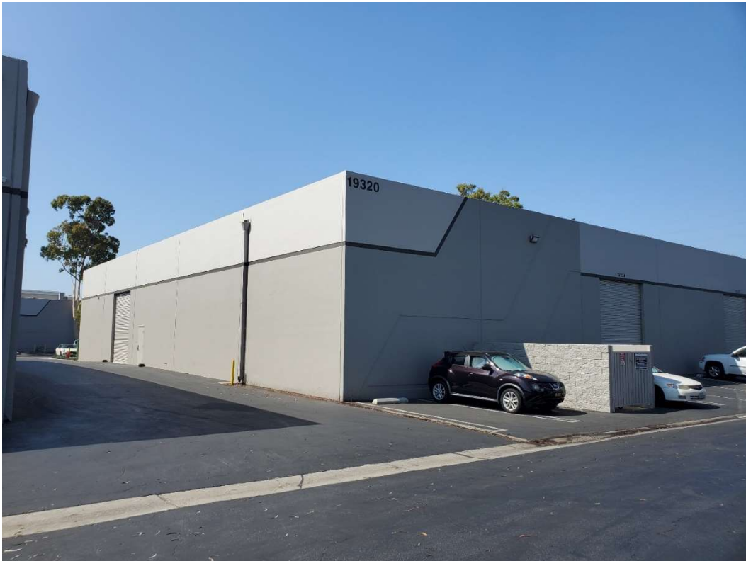
Figure 5-22. 19320 Van Ness Avenue rear (eastern) elevation, facing southwest.
