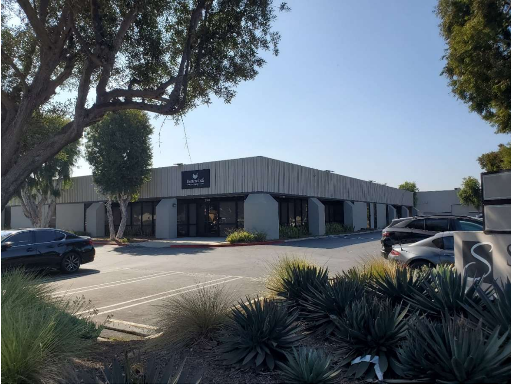
Figure 5-1. 2150 West 190th Street, primary (northwestern) elevation, facing southwest.
