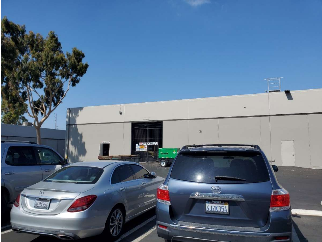
Figure 5-20. 19260 Van Ness Avenue rear (eastern) elevation, facing west.
