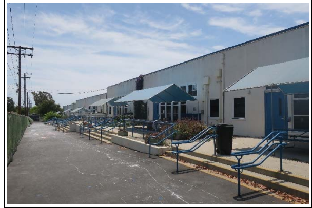
Building F, east façade, view south (ARG, 2021)
