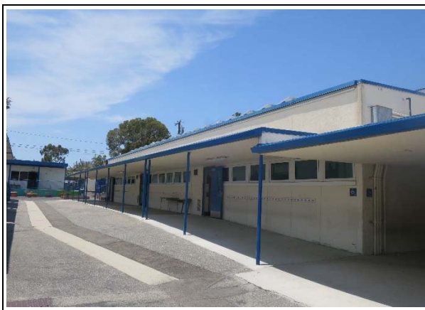
Building D, south façade, view northwest (ARG, 2021)
