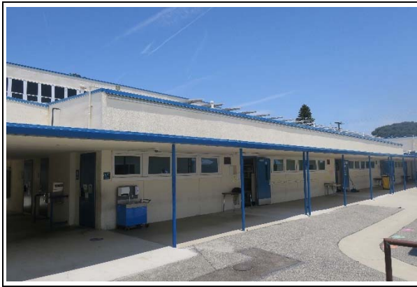
Building E, south façade, view northeast (ARG, 2021)
