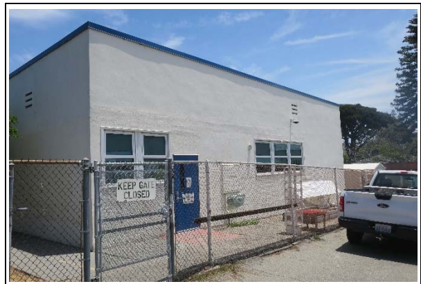
Building G, west façade as seen from 24 th Place, view east (ARG, 2021)
