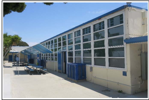
Building E, north façade, view east (ARG, 2021)
