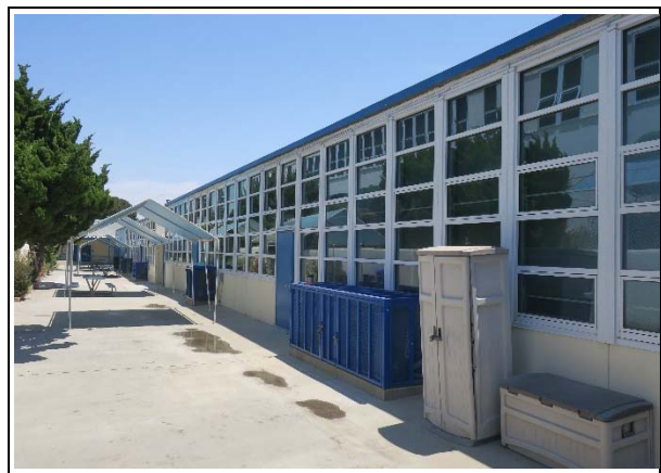
Building D, north façade, view east (ARG, 2021)
