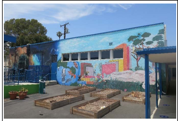
Building C, south façade, view northwest (ARG, 2021)
