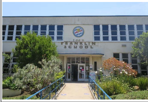
Building B, primary (north) façade, view southeast (ARG, 2021)
