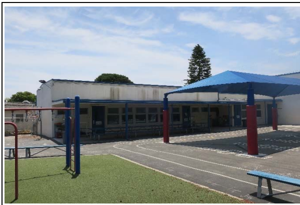
Building G, north façade, view southwest (ARG, 2021)
