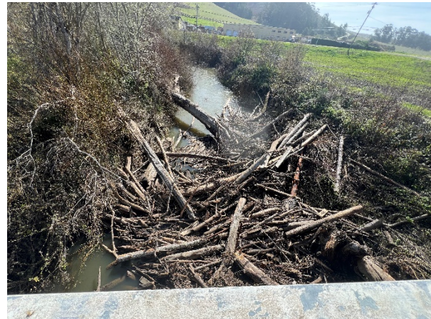
Photo 1. Pescadero Creek Bridge, facing upstream (2/18/2025).
