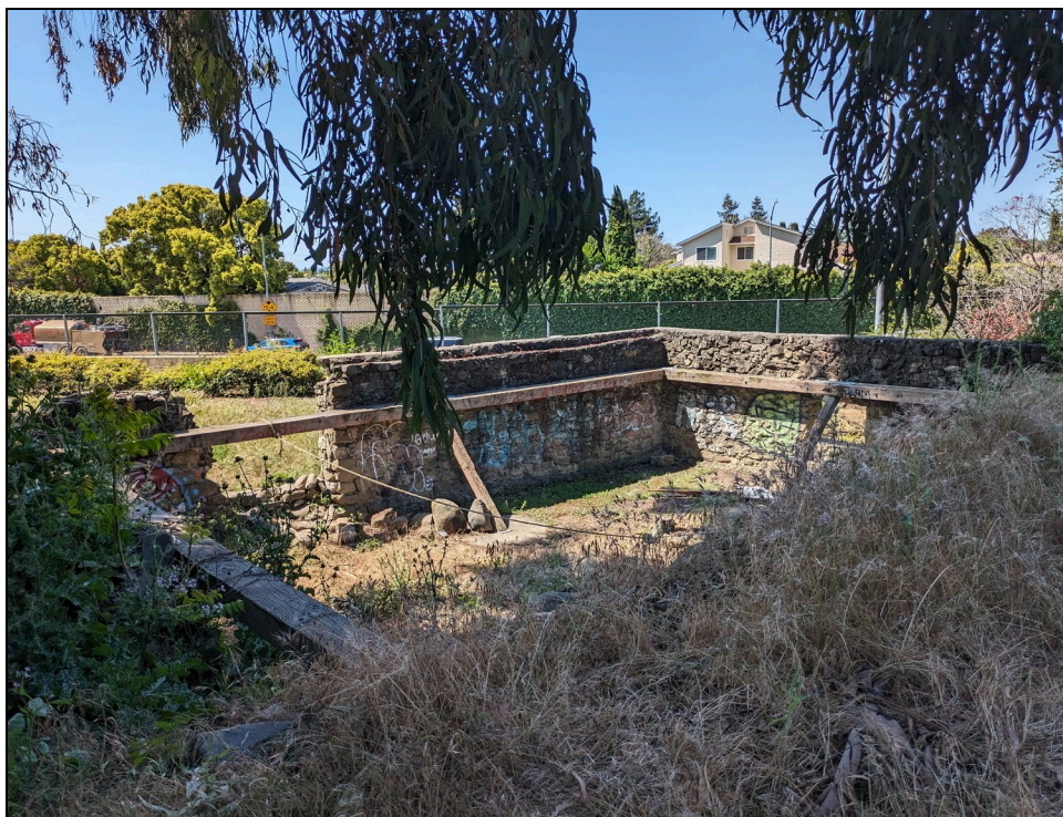
Figure 9. Interior view of the southwest corner of Feature 1, facing southwest.
