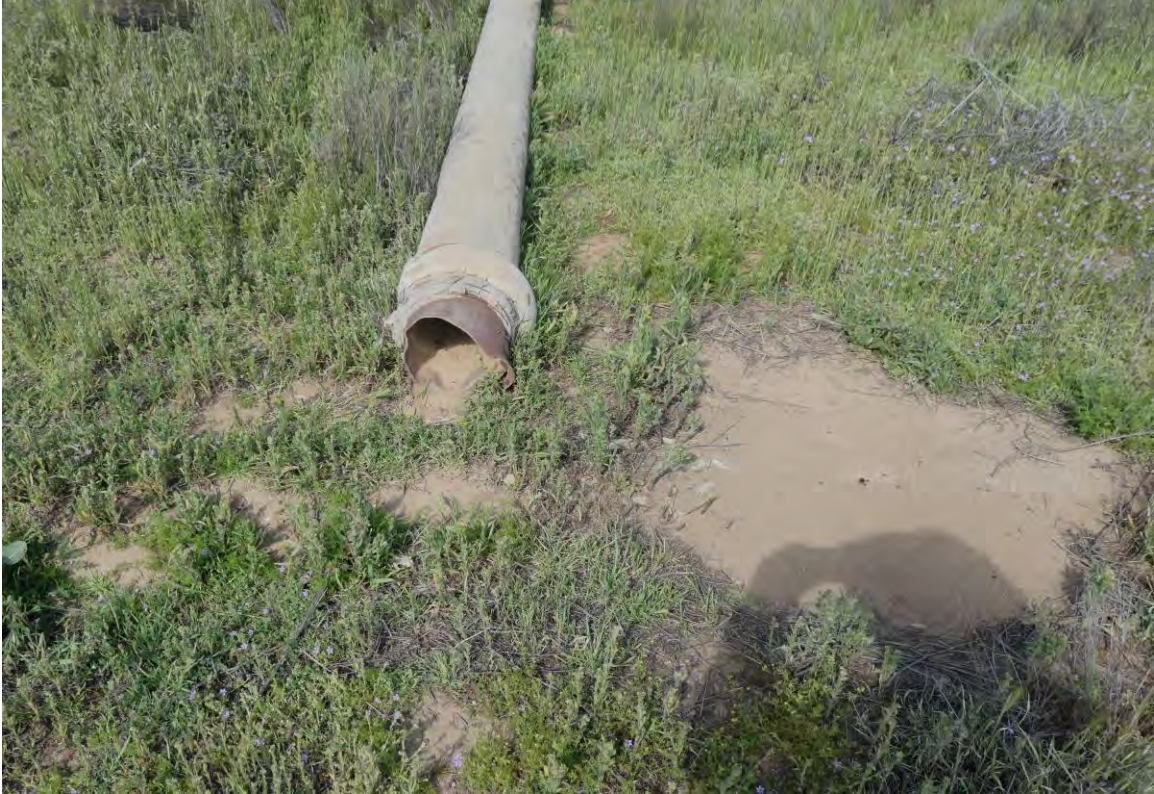
Photograph 9: One of the potential owl burrows and old pipe both occupied by ground squirrels, March 2024.
